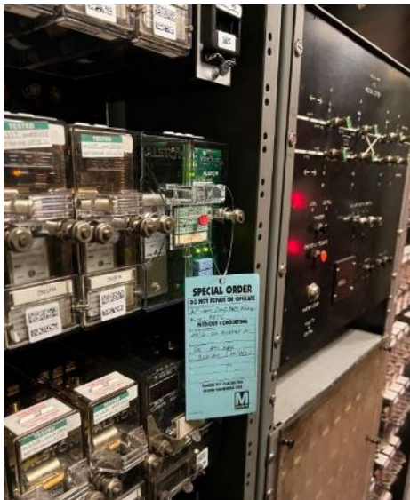
Vital Relays and Local Control Panel
