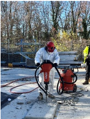
Electric jackhammer demonstration
