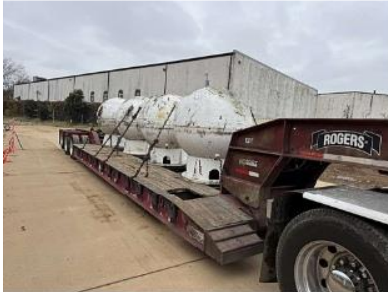
Removal & Haul-out of Underground Storage Tanks (USTs)
