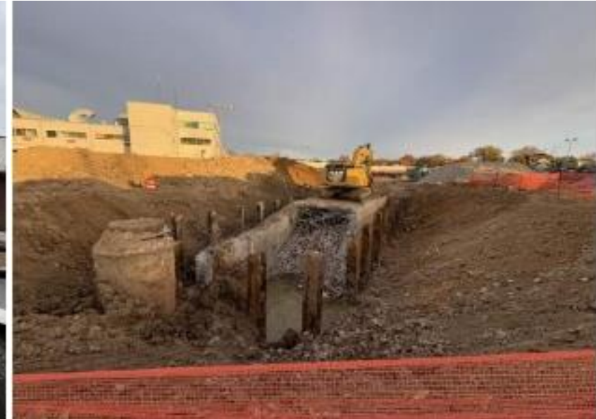
Demolition of Underground Stormwater Retention Tanks
