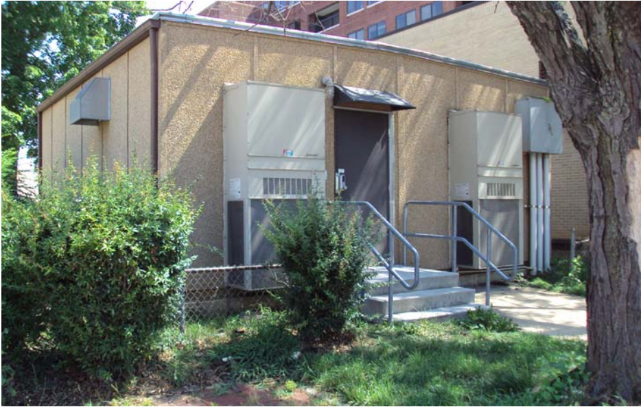
Photo 17 - EDR Site 4 - former site of Virginia Rug Cleaning Corp
