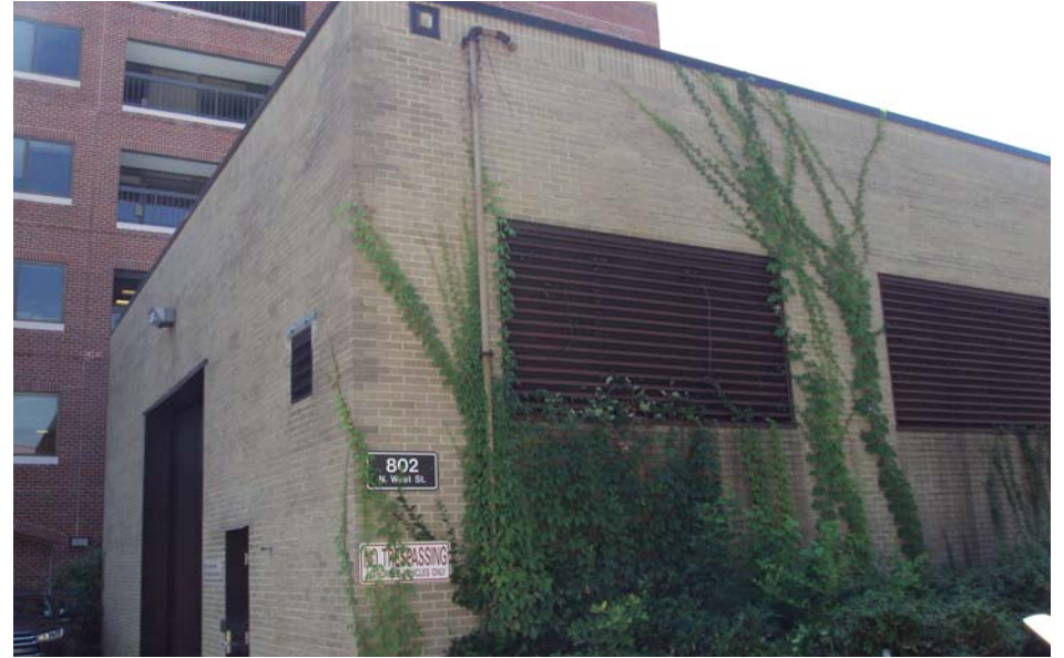
Photo 10 - C12 Traction Power Substation with vent pipe
