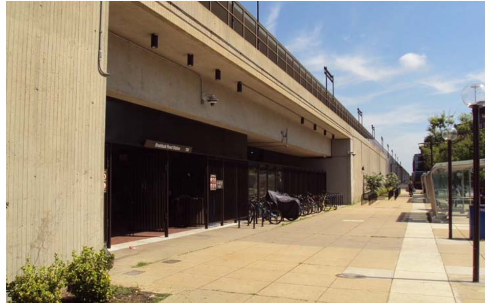
Photo 02 - Braddock Road Metro Station Entrance
