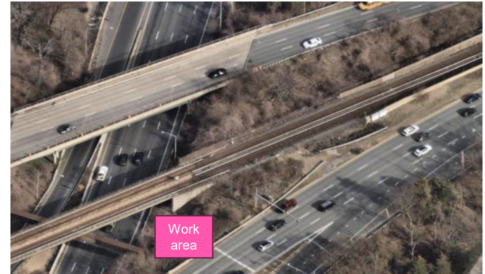
Grosvenor Aerial Structure Maintenance
