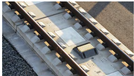
CBTC wayside equipment
