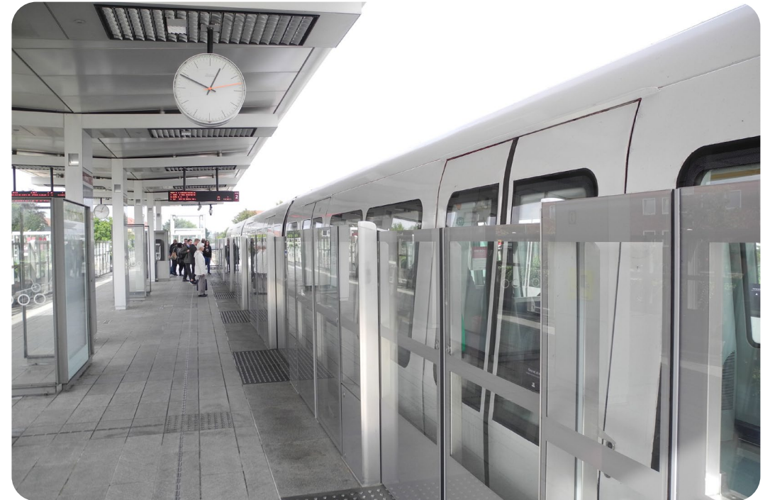
Kastrup Station (Copenhagen Metro), with platform doors – 2015
