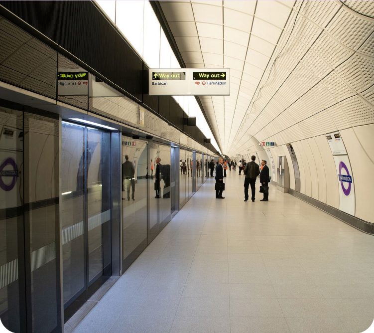
Transport for London: Elizabeth Line Trackway completely enclosed
