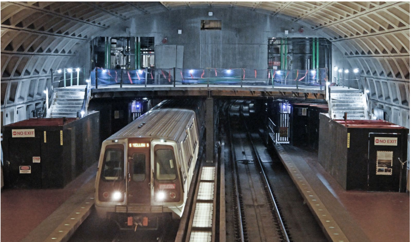
Pictured: Construction on the new Crystal City Metro station entrance
