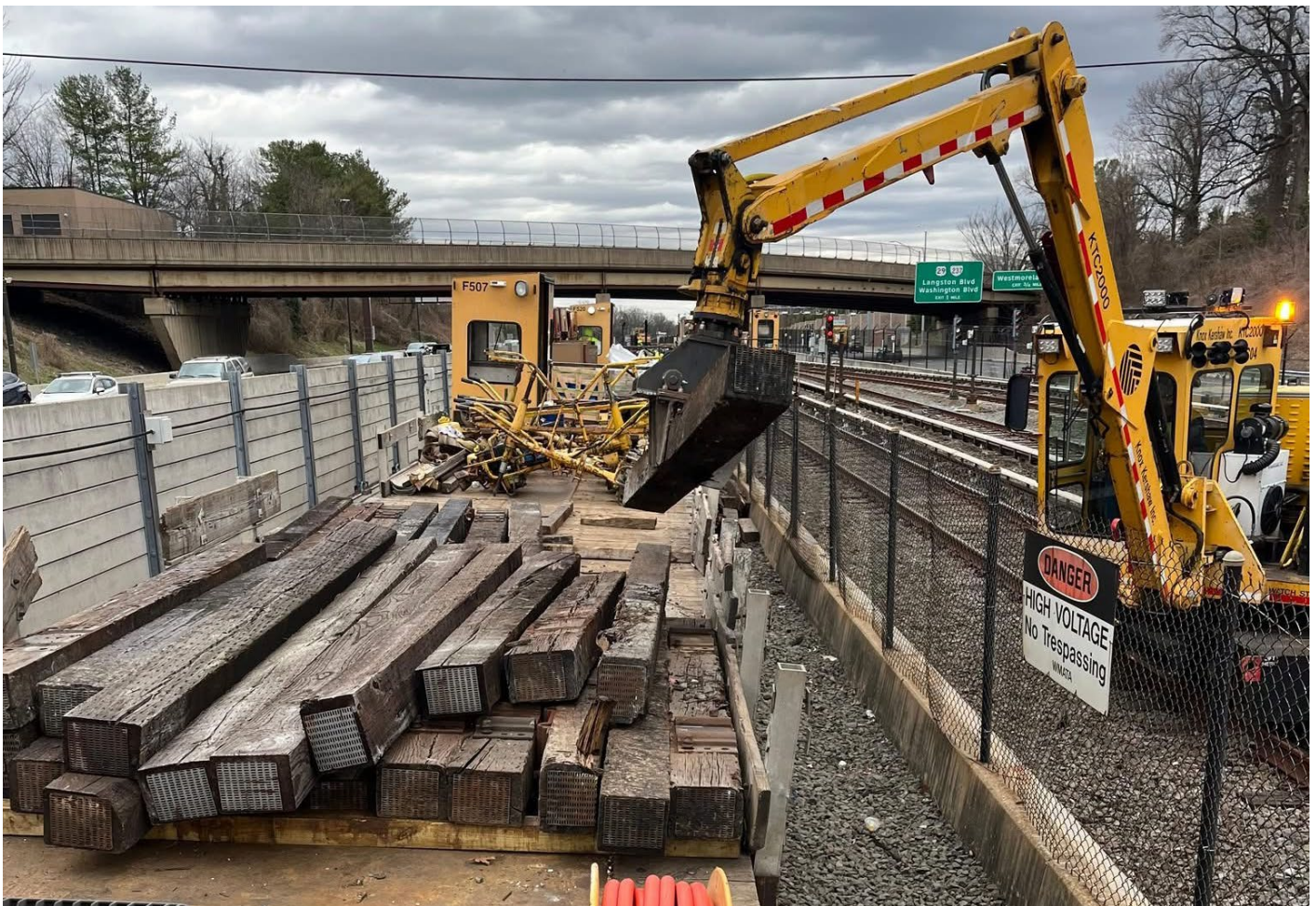
Pictured: Metro Rail preventive track maintenance
