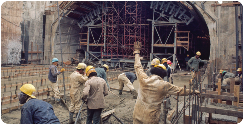
Union Station Under Construction, circa 1974
