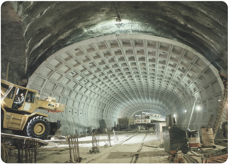
Dupont Circle Construction, 1975
