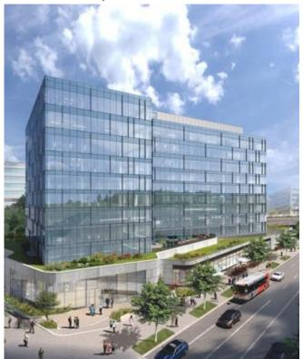
METRO ACQUIRED 300 7<sup>TH</sup> STREET IN 2018 AND SELECTED JAIR LYNCH REAL ESTATE TO MANAGE THE DEVELOPMENT AND MODERNIZATION OF 8-STORY CAST-IN-PLACE CONCRETE BUILDING INTO CLASS A COMMERCIAL BUILDING WITH ADDITION OF THREE STEEL FRAME FLOORS AND GROUND FLOOR PODIUM, TOTALING 290,00 SQUARE FEET.
