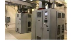
maintainability. These generators range from 50kW to 600kW and are connected to various Metro's electrical systems, including Stations, Parking and Bus Garages.
