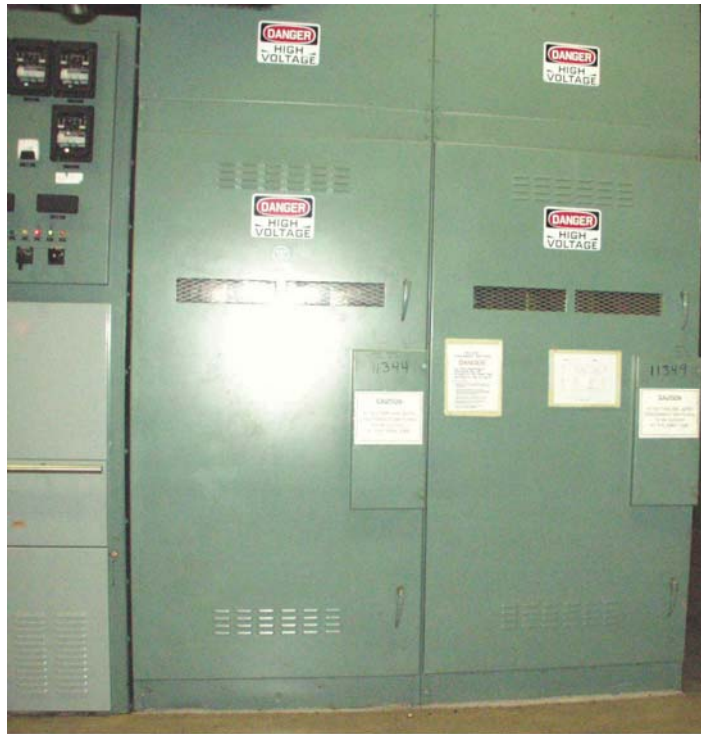
Fig. 1 WESTINGHOUSE 34.5KV LOAD INTERRUPTER SWITCH TYPE WLI
