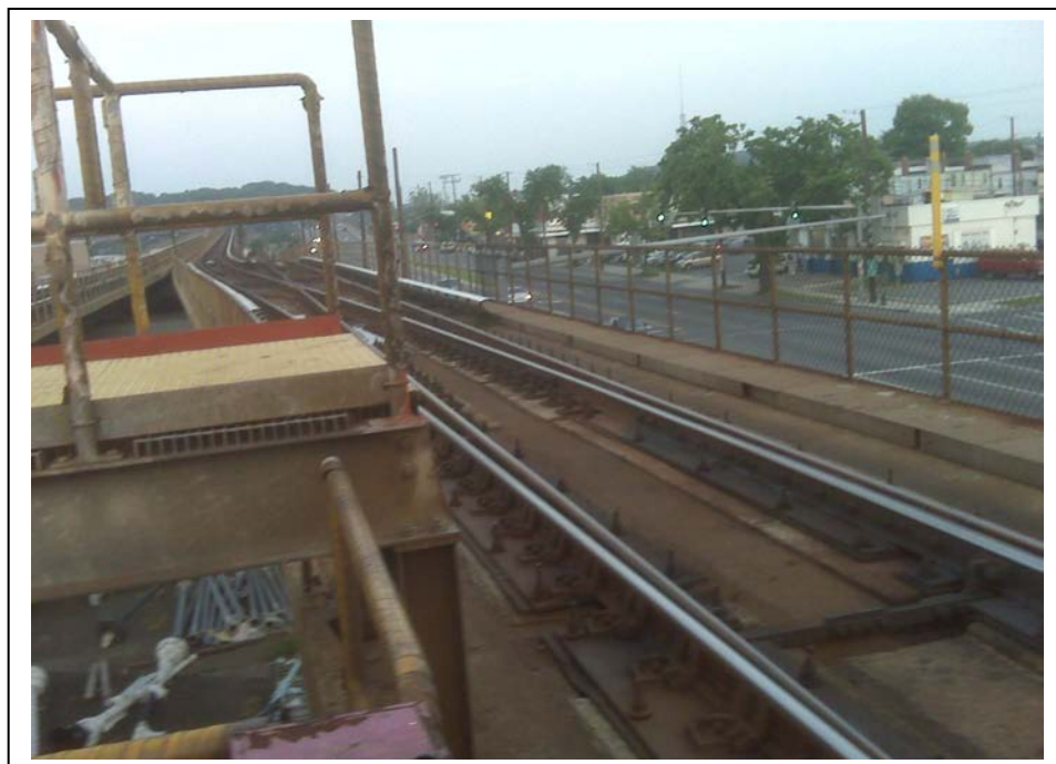
Picture 4 - D & G Platform, Track 1
