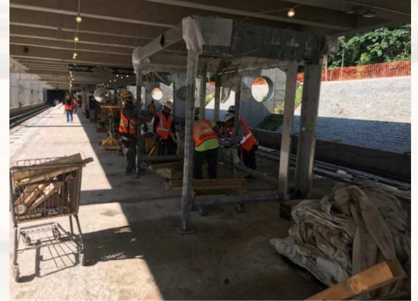
Installing new windscreens at Huntington Station
