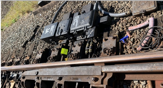
Signaling Switch Machine Replacement
