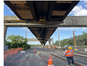
Track and Structures Rehabilitation
