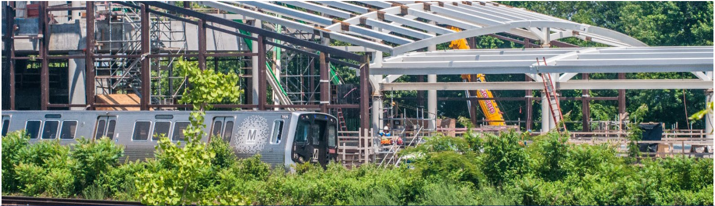
Metrorail train passing by Potomac Yard Station construction
