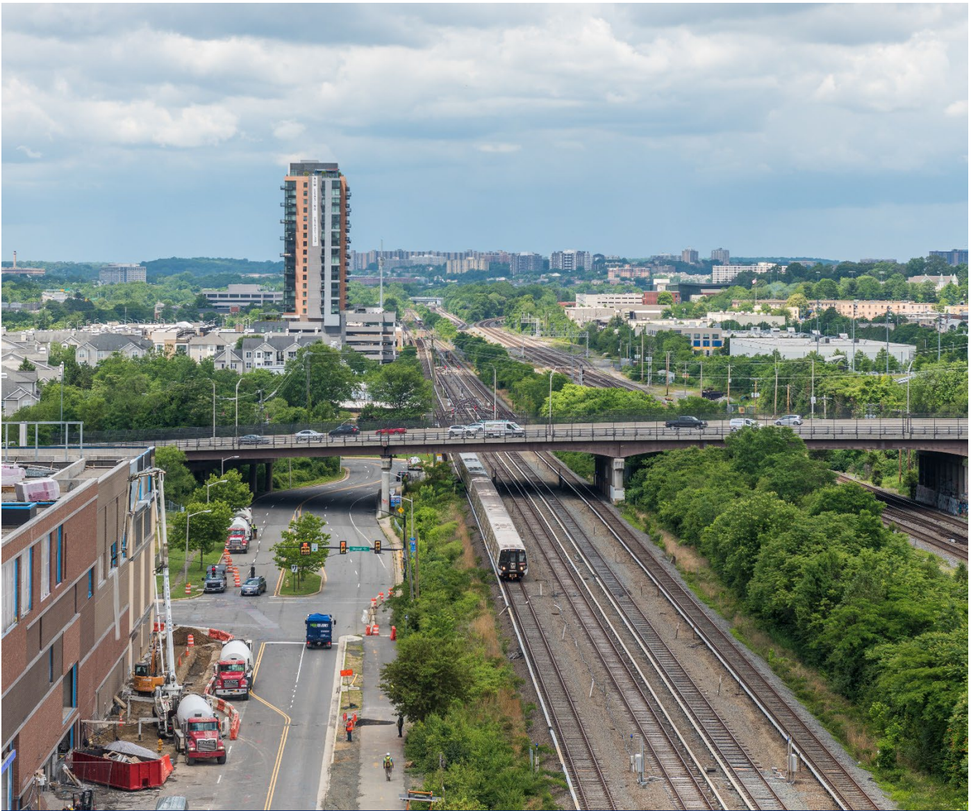
Construction for new Metro office and larger redevelopment near Eisenhower Ave Station
