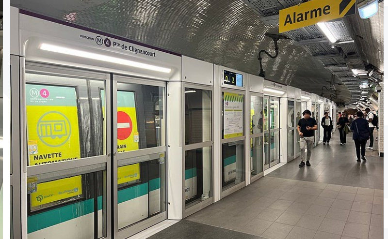
Paris Metro: Line 4 Platform Screen Door Testing
