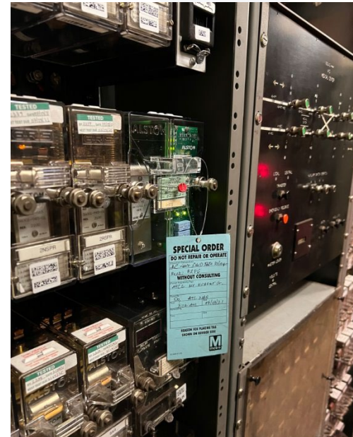
Vital Relays and Local Control Panel
