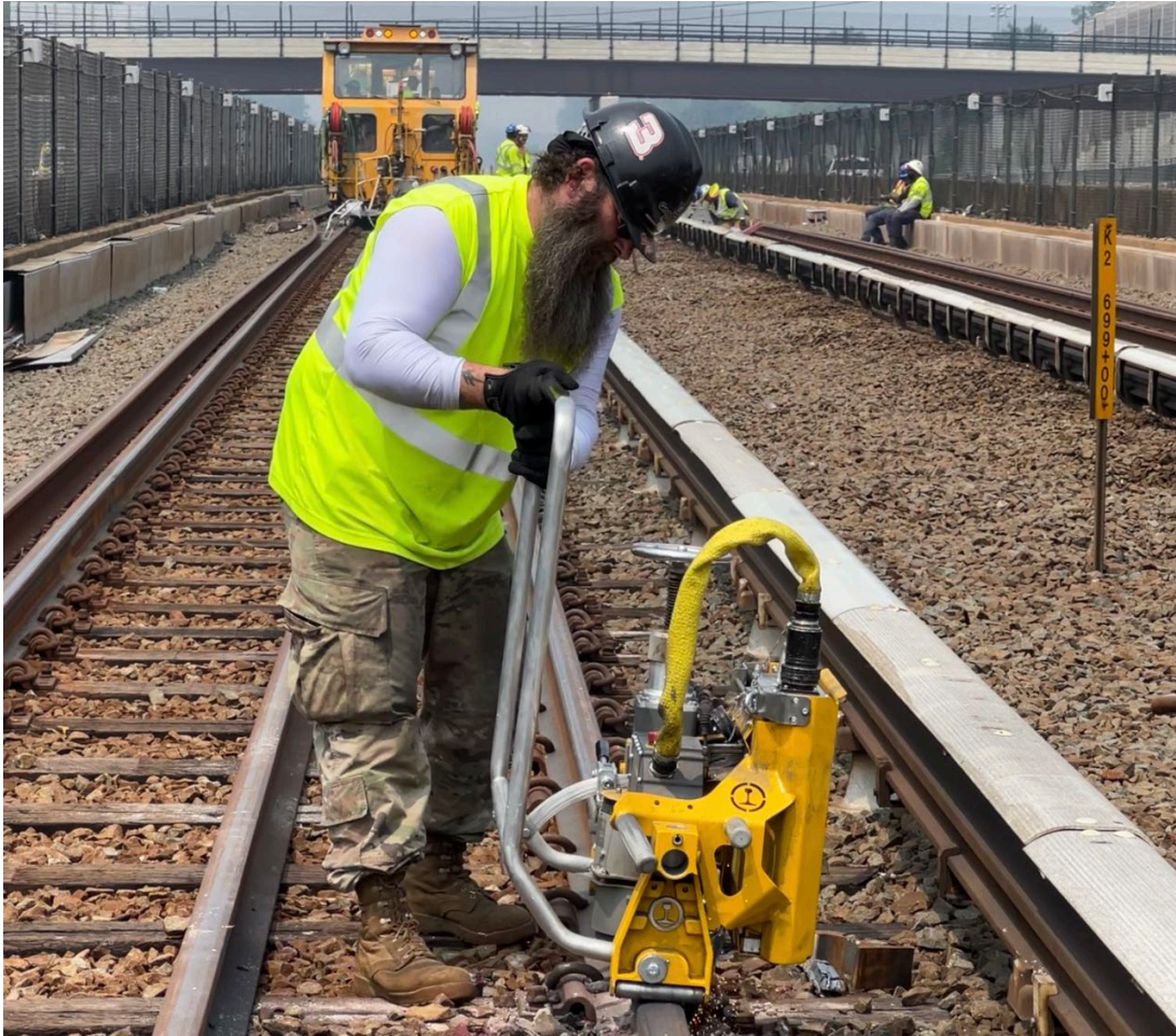
Battery-powered rail surface grinder (K-Line shutdown, summer 2023)
