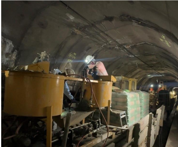
Water Leak Mitigation on Red Line
