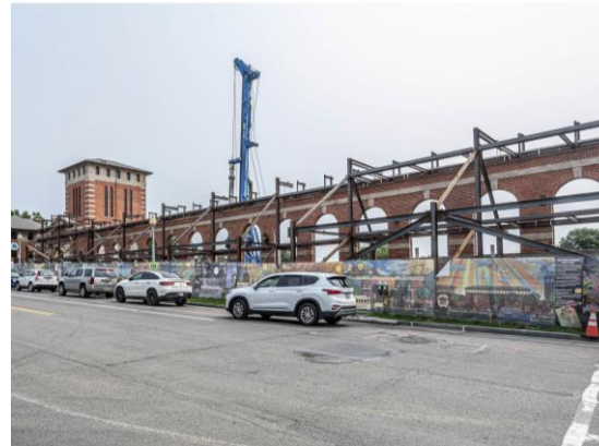
Historical Façade/Tower Bracing & Monitoring
