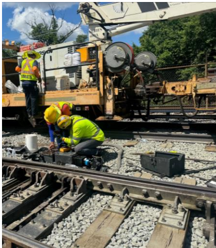
Switch Machine Replacement at Takoma
