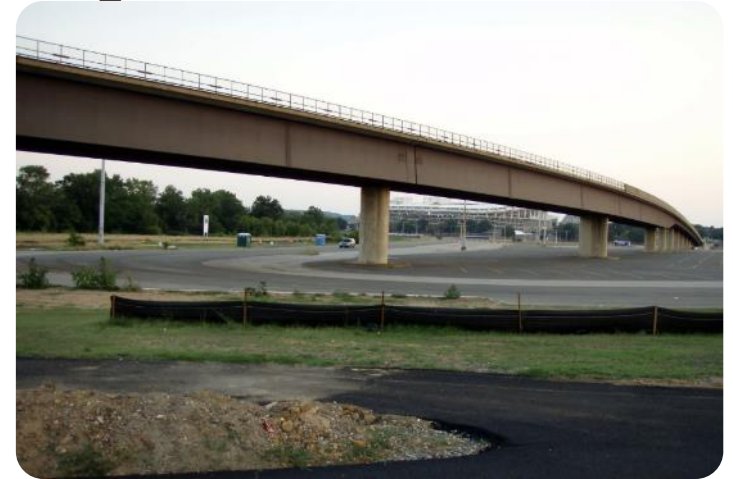
Aerial tracks east of Stadium-Armory Station
