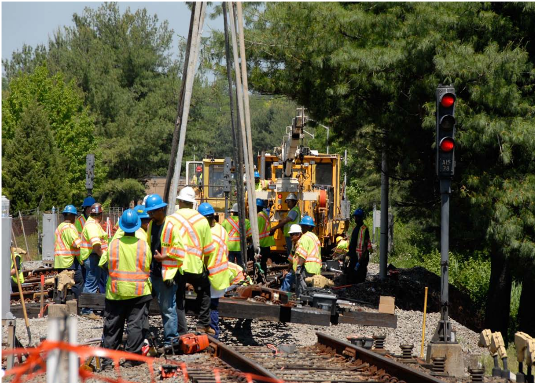
Photo of track work at Shady Grove
