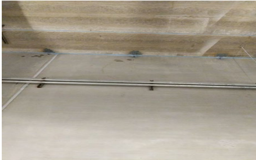
Herndon: Figure 11: Efflorescence at Panel 2538. Source: DeSimone
