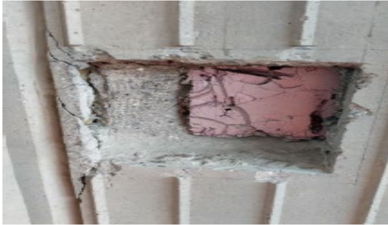
Ashburn: Figure 8: Piece of precast concrete panel cut-out at panel 5125. Source: DeSimone
