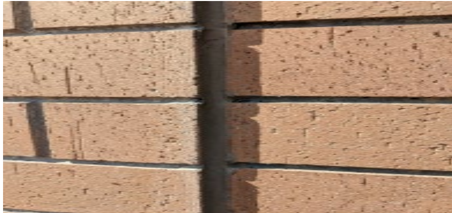
Innovation: Figure 7: Edge of panel outboard and not flush with adjacent panel at Panels 200, 201. Source: DeSimone
