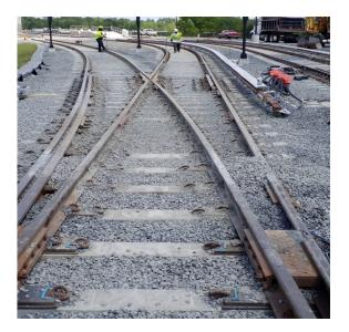
On August 12, 2019 the OIG team met with the WMATA Project staff and contract Subject Matter Expert co-located at the Rail Yard. The staff and technical advisor expressed specific concerns about the chronic failures of turnouts (#8) failing to meet required track geometry standards and exhibiting 'tight gage' conditions.
