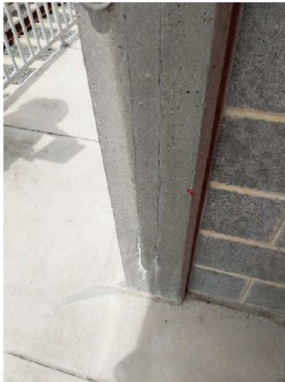
Figure 42: Exterior face of Panel WP-1313. Refer to Appendix C for photo showing location of cracking at previous repair. Source: DeSimone.
