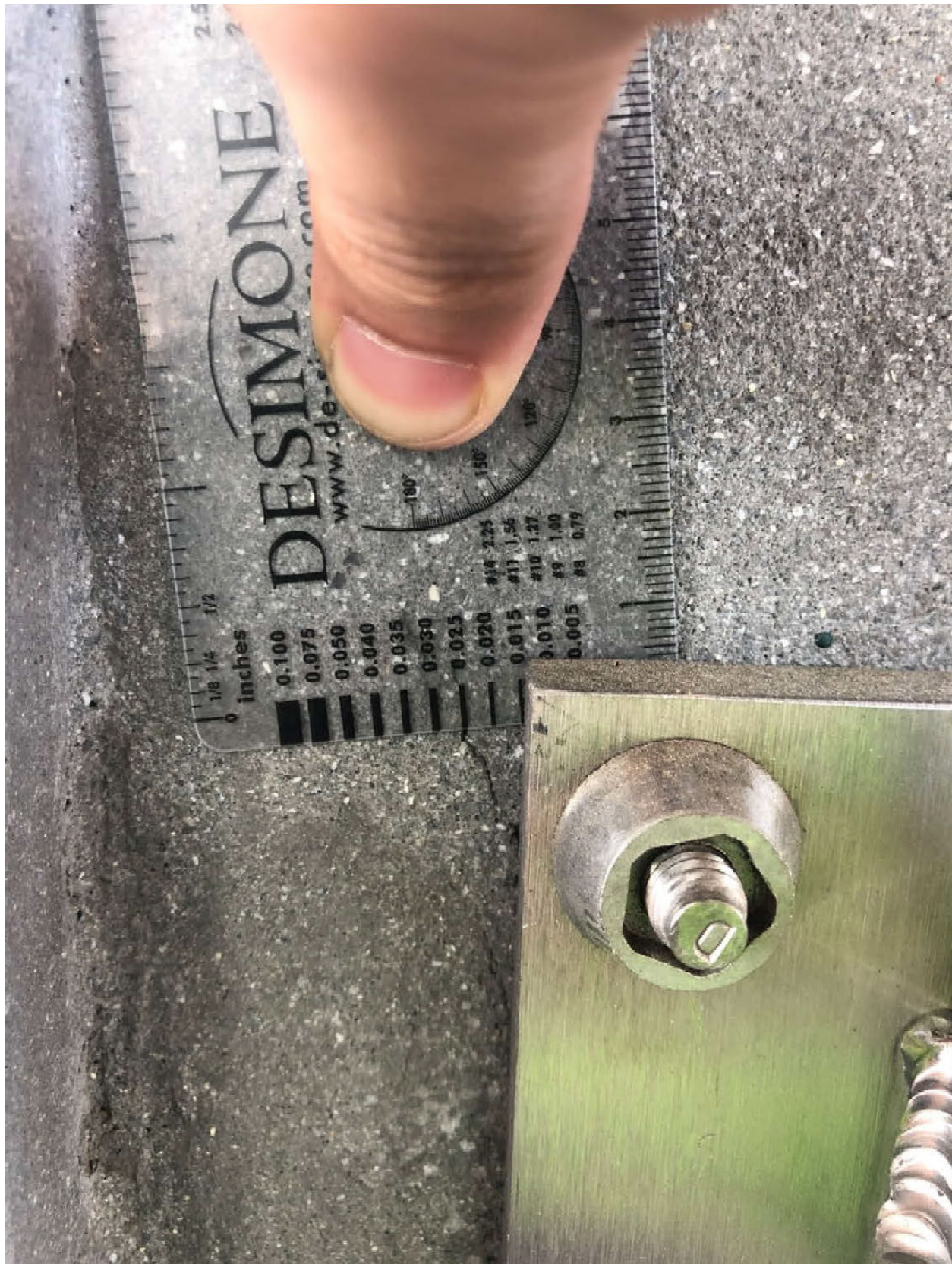
Figure 46: Crack at interior face of Panel WP-1233. Source: DeSimone.
