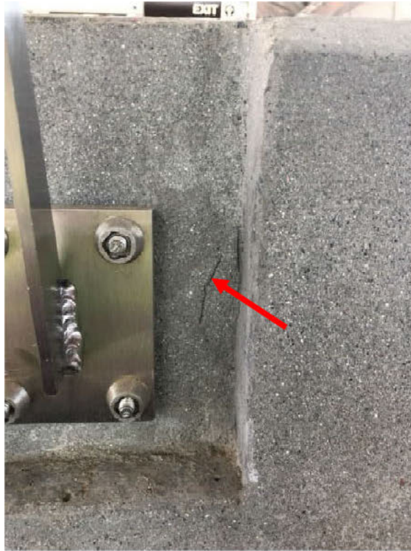
Figure 49: Interior face of Panel WP-1233. Source: DeSimone.
