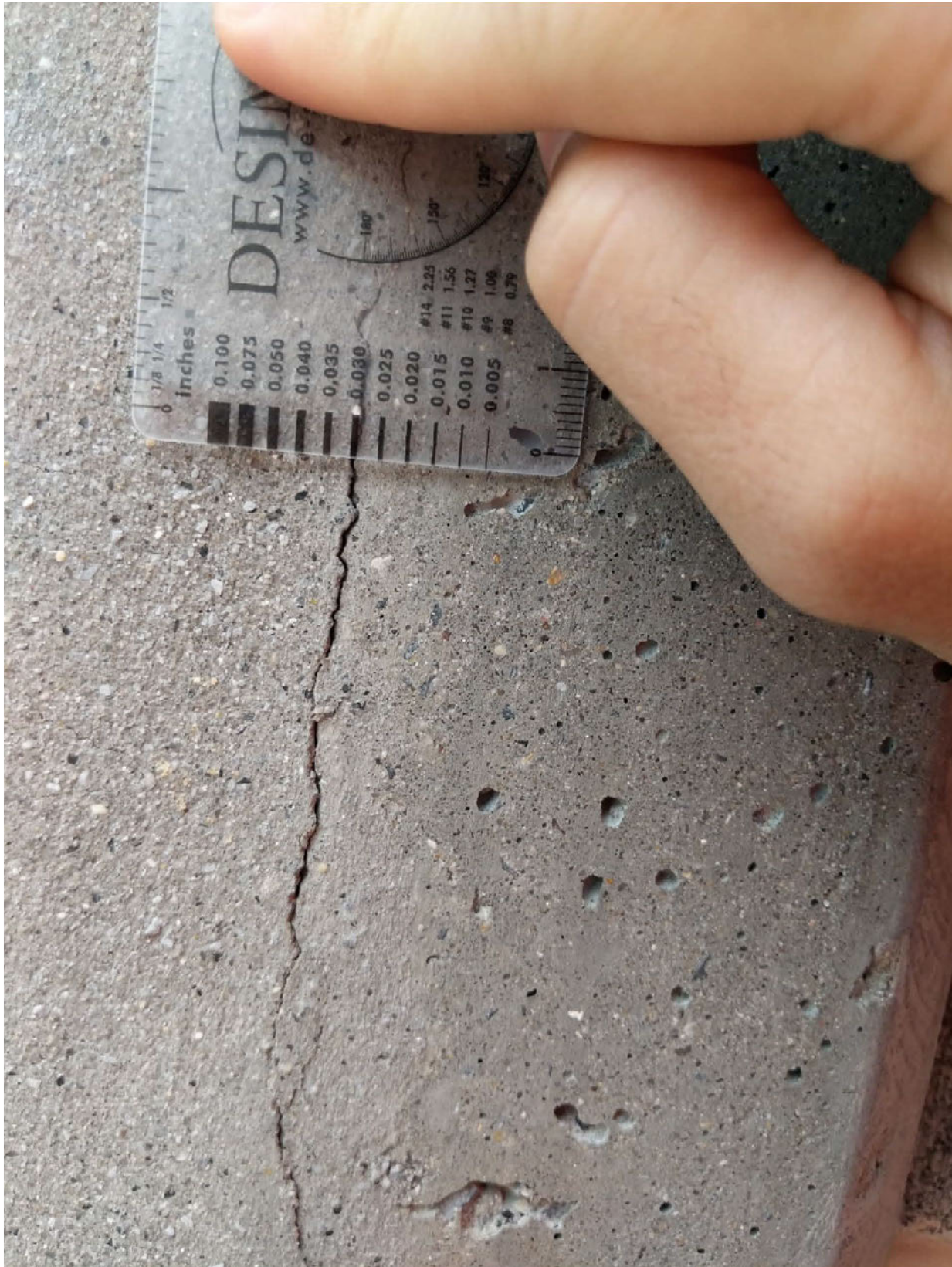
Figure 40: Crack at previous repair location at exterior face of Panel WP-1313. Source: DeSimone.
