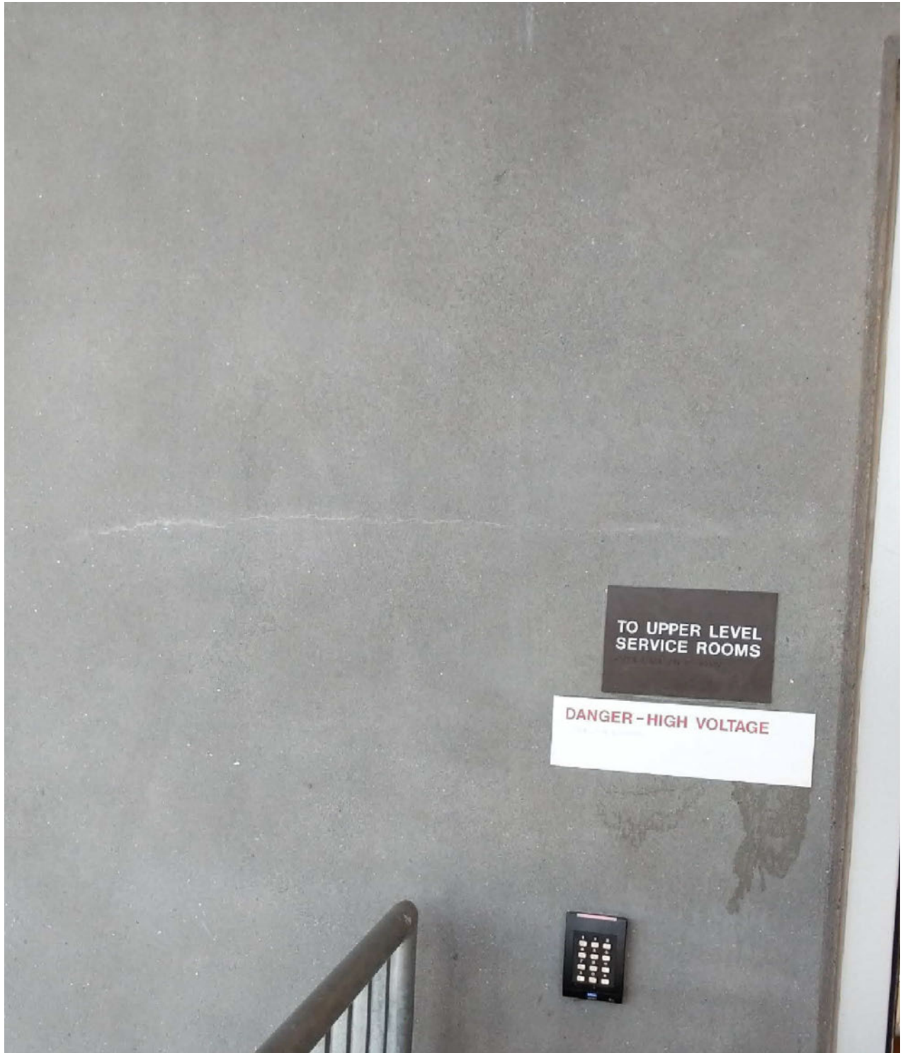
Figure 10: Repaired crack at exterior of Panel 232. Source: DeSimone
