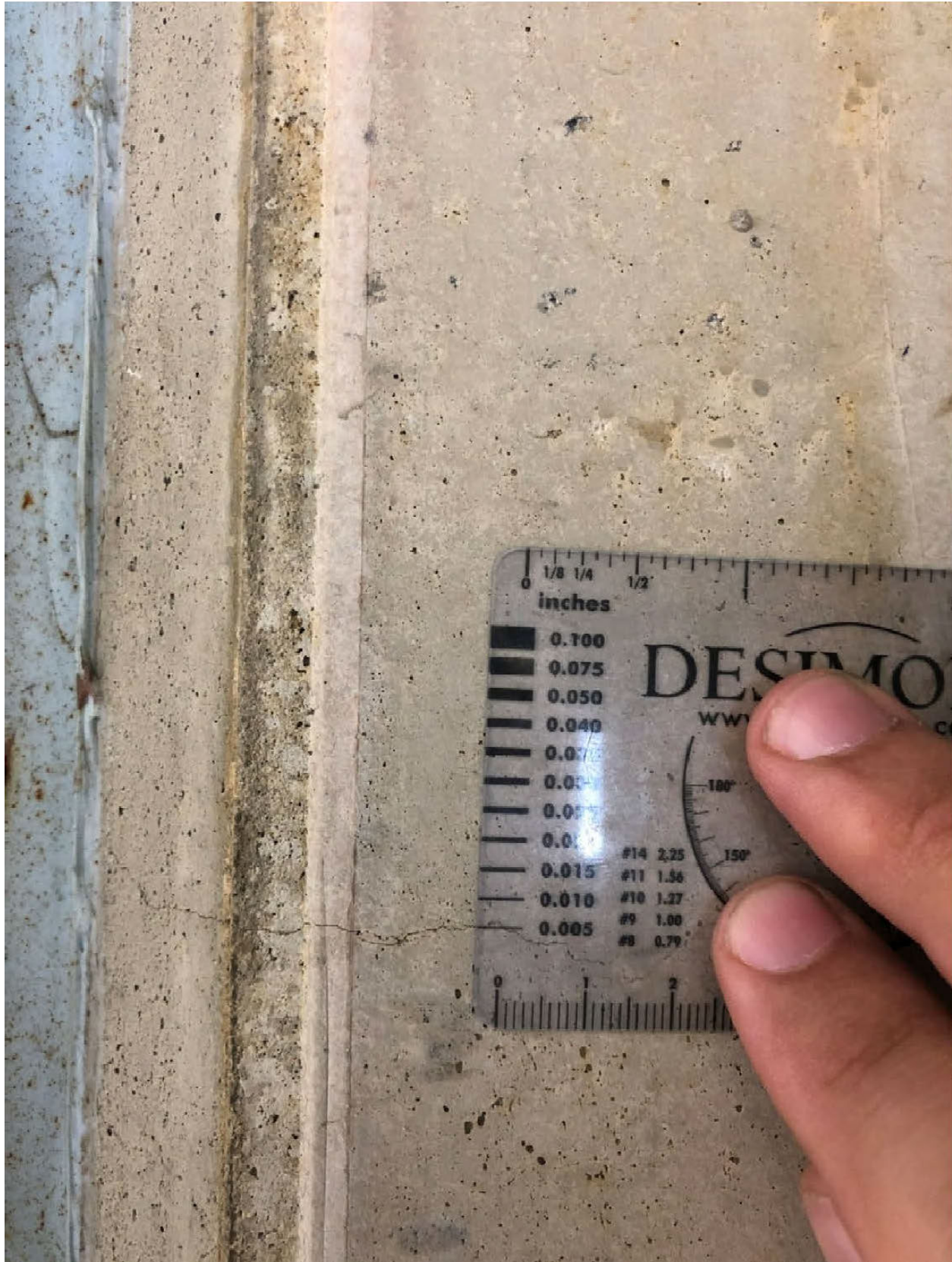
Figure 23: Crack at interior face of Panel 1421. Source: DeSimone.
