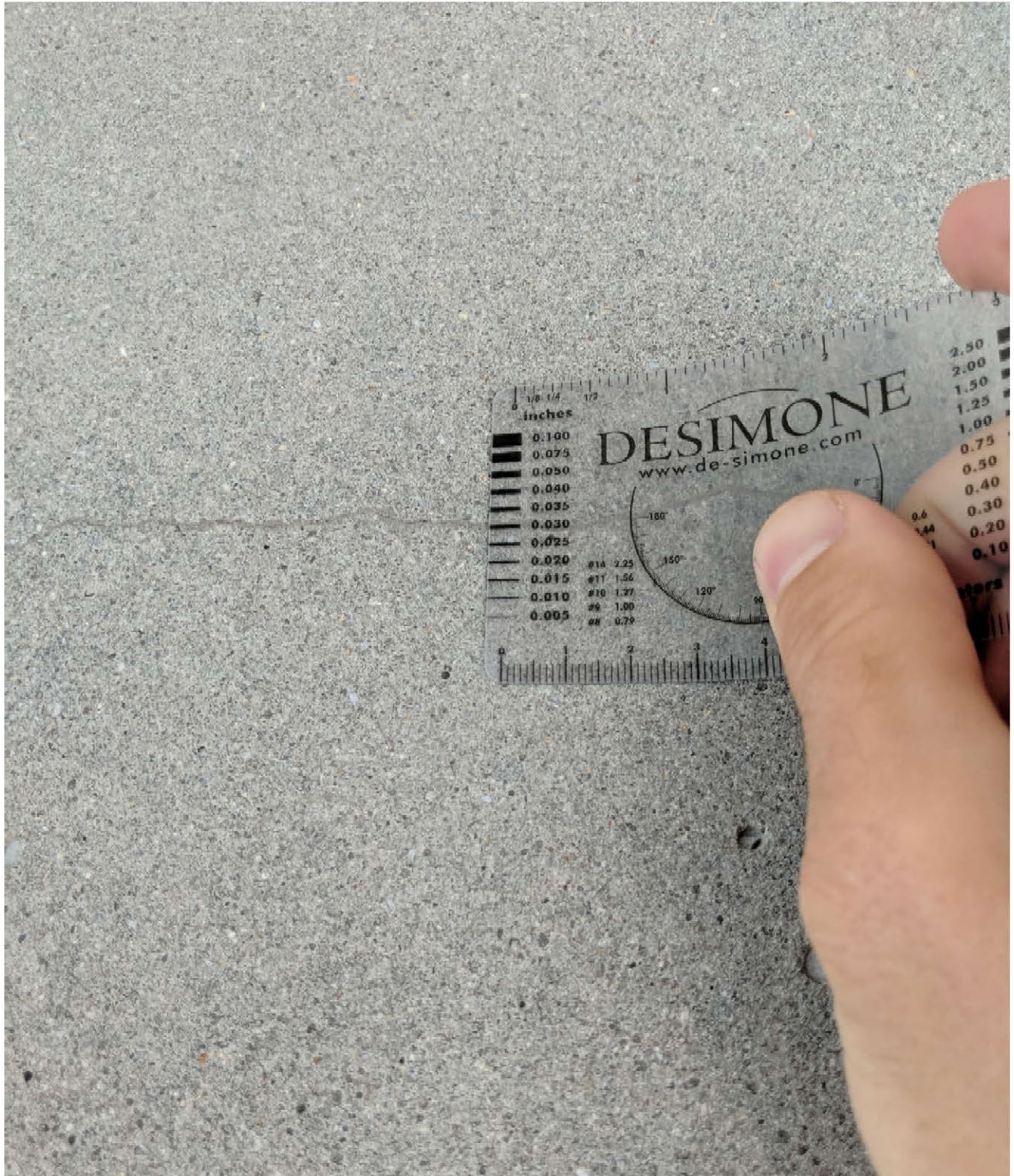
Figure 15: Repaired crack at exterior face of Panel 402. Source: DeSimone.
