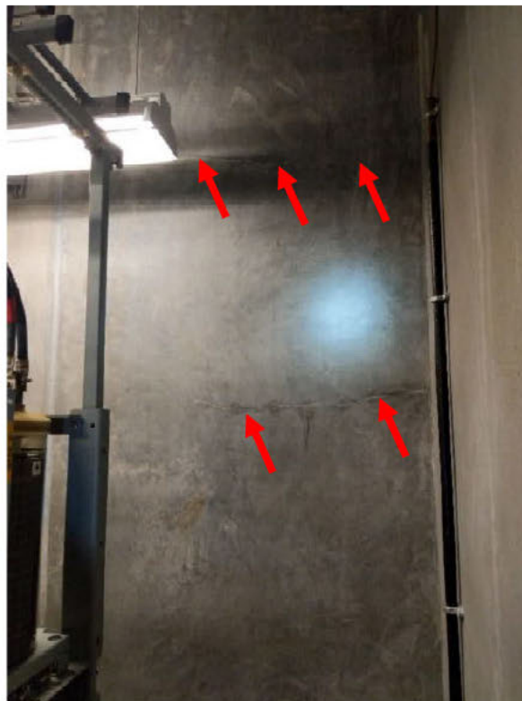
Figure 16: Interior face of Panel 206. Refer to Appendix C for photo showing location of cracking at previous repair. Source: DeSimone.
