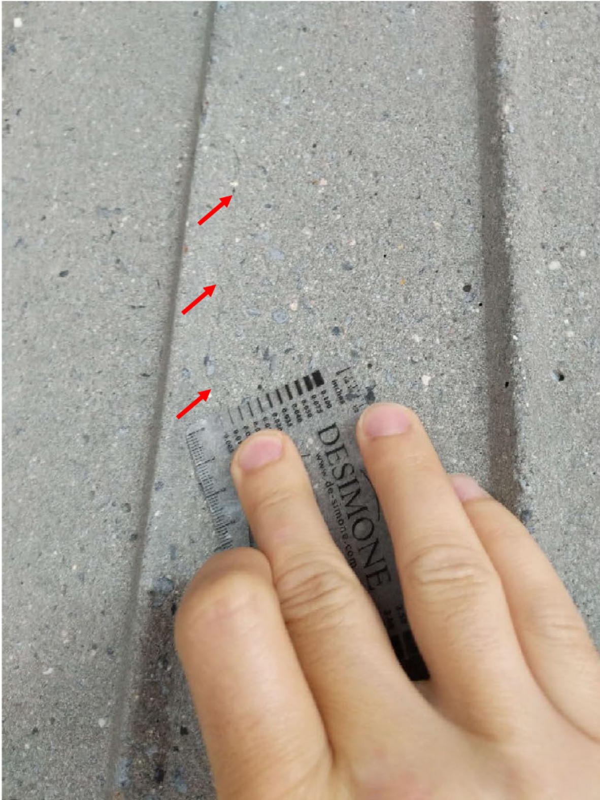
Figure 7: Crack at ticketing booth side of Panel 100. Source: DeSimone.
