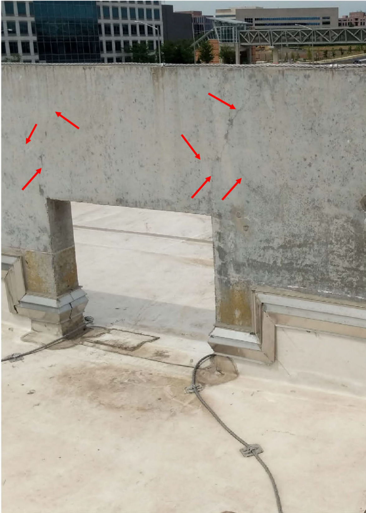
Figure 42: Spider cracks at interior face of Panel WP-1324. Source: DeSimone.
