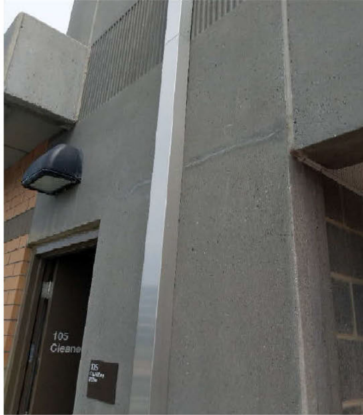
Figure 3: Typical Exterior Precast Concrete Panel. Source: DeSimone
