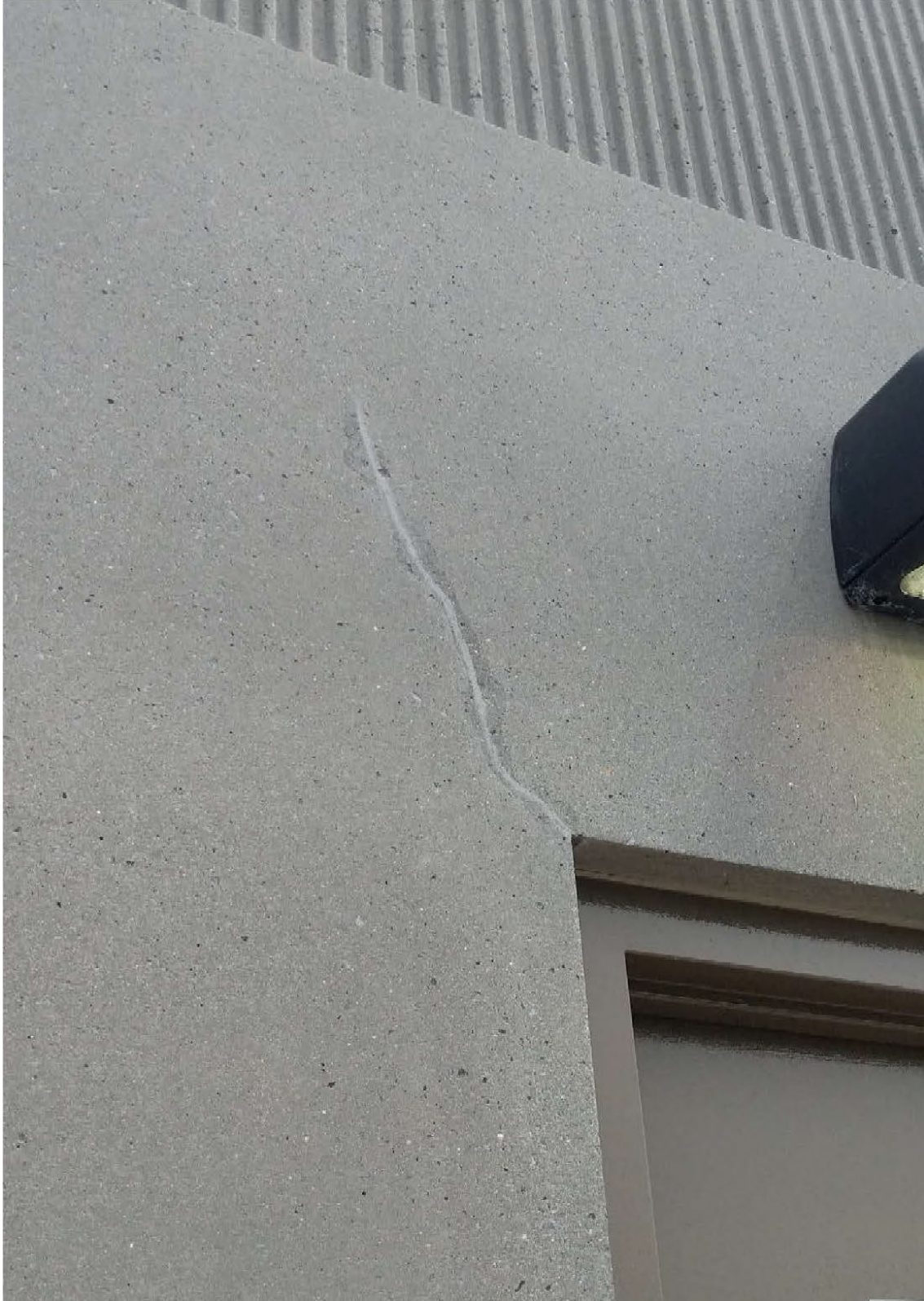
Figure 41: Previously repaired crack at exterior face of Panel WP-1315. Source: DeSimone.
