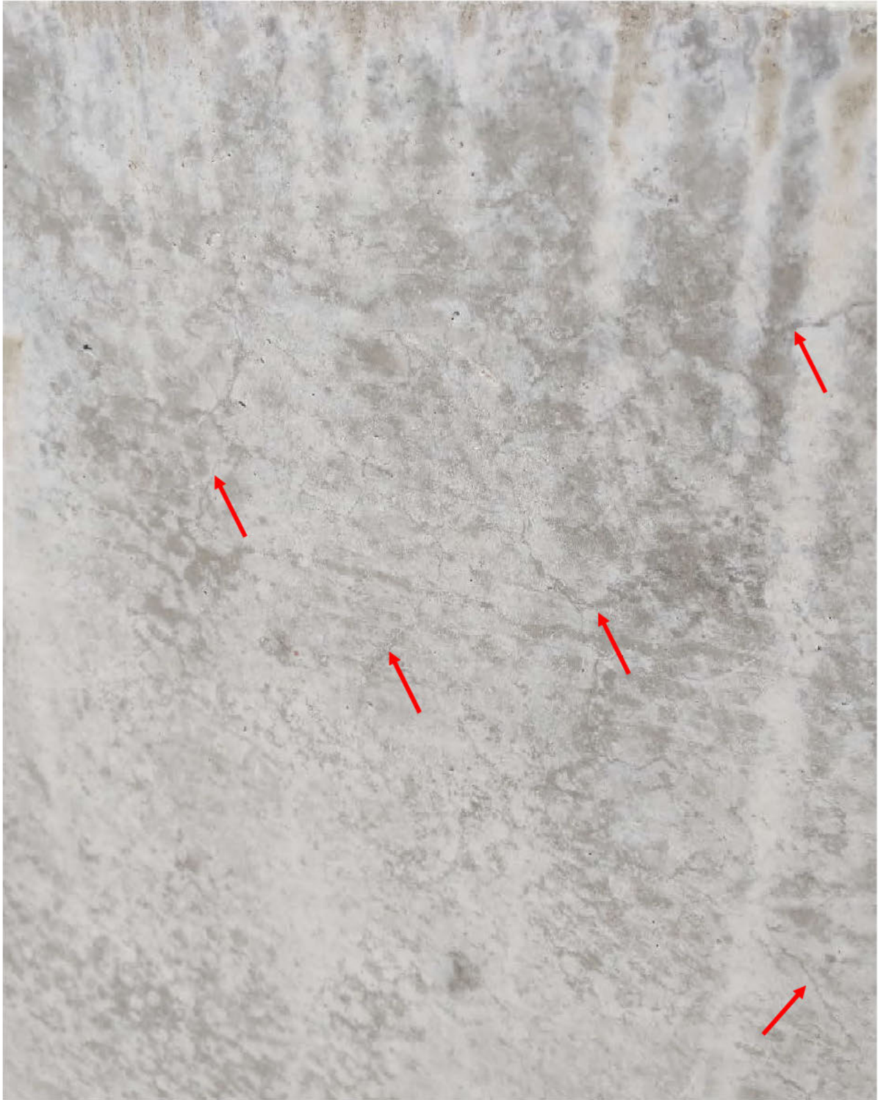
Figure 37: Spider cracks at interior of Panel WP-1321-RI. Source: DeSimone.
