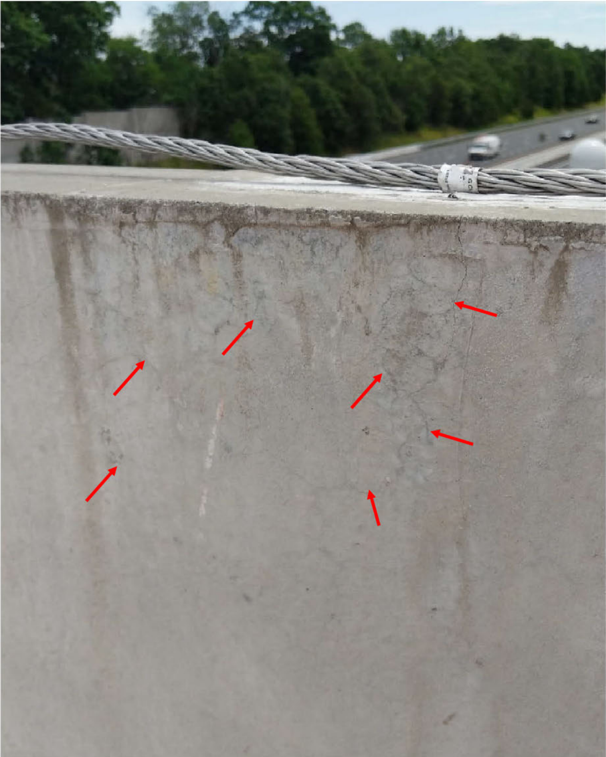
Figure 43: Spider cracks at interior face of Panel WP-1329. Source: DeSimone.
