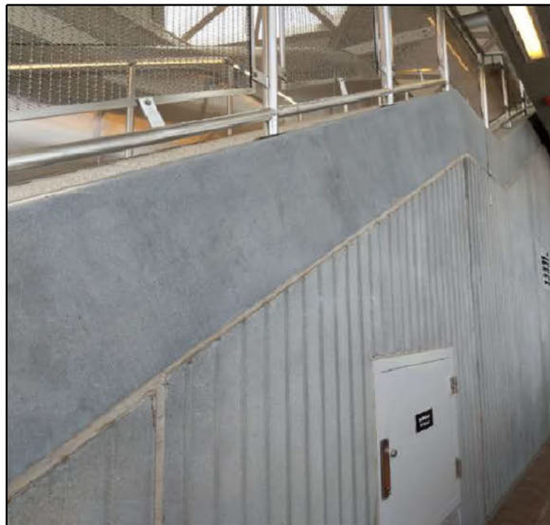
Figure 4: Typical Stair Precast Concrete Element. Source: DeSimone.
