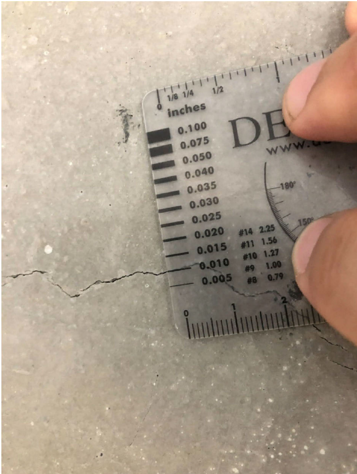
Figure 33: Crack at interior face of Panel 1904. Source: DeSimone.
