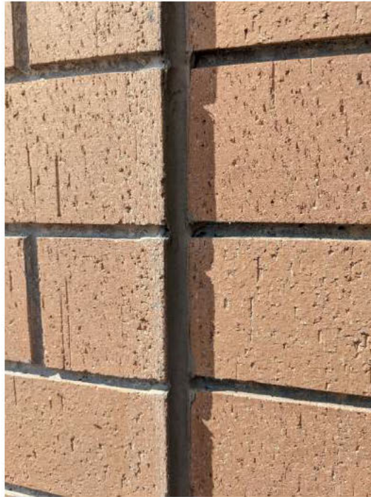
Figure 7: Edge of panel outboard and not flush with adjacent panel at Panels 200, 201. Source: DeSimone.
