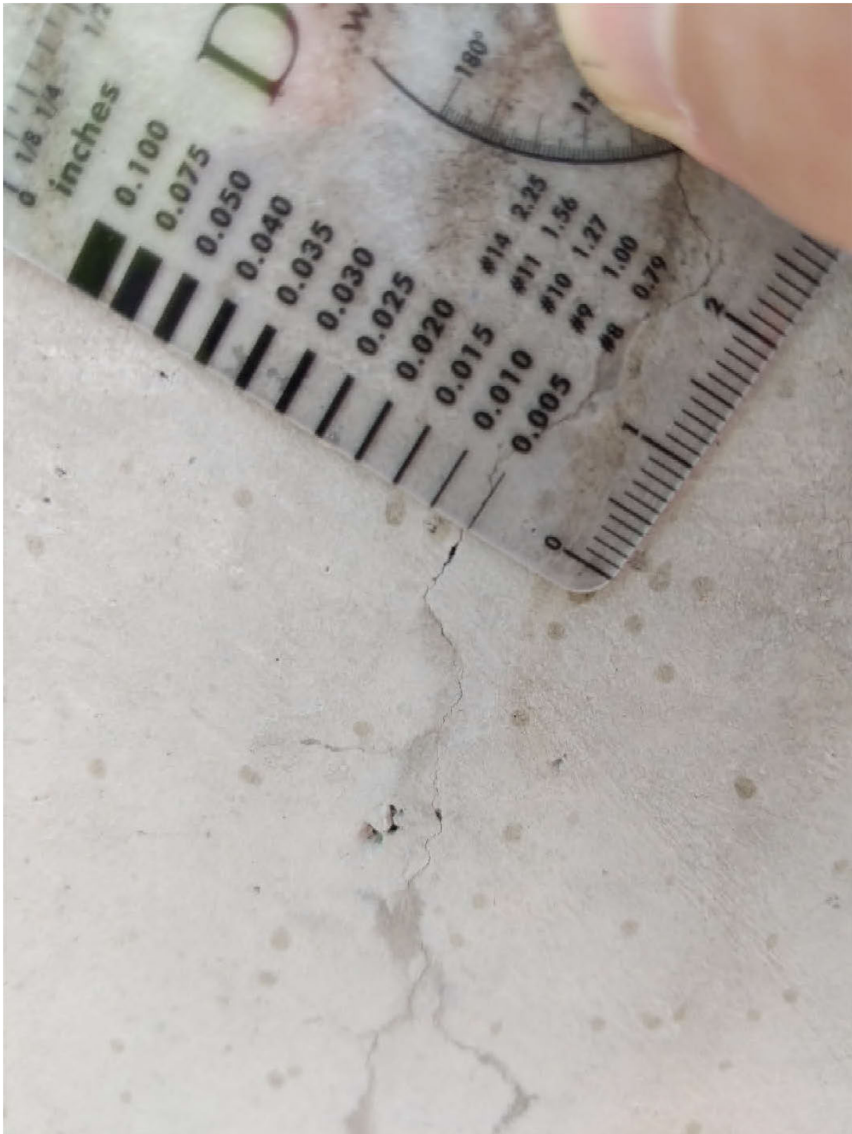
Figure 36: Crack at Interior face of Panel WP-1328-R!. Source: DeSimone.
