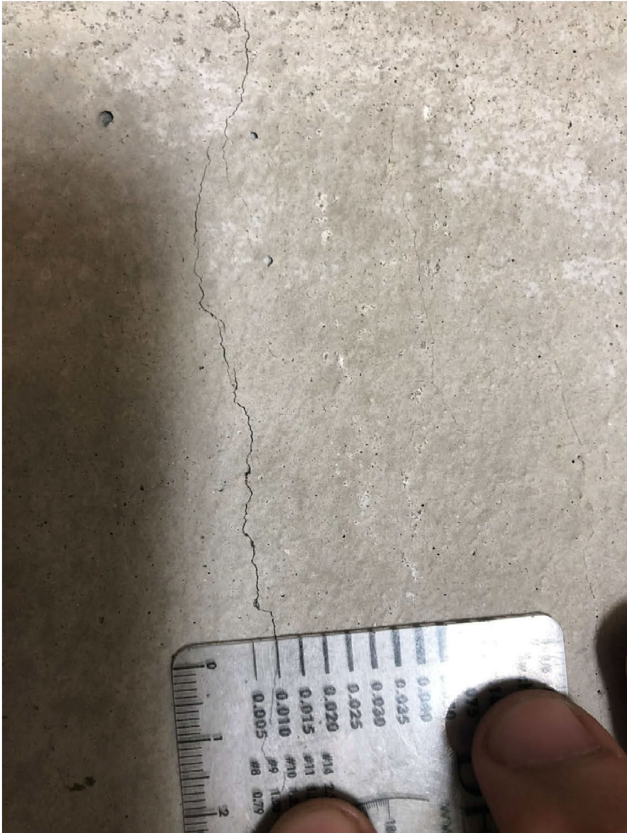
Figure 28: Crack at Interior face of Panel 1904. Source: DeSimone.
