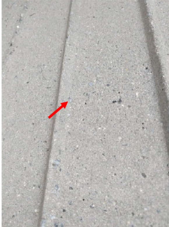
Figure 11: Crack at ticketing booth side of Panel 100. Source: DeSimone
