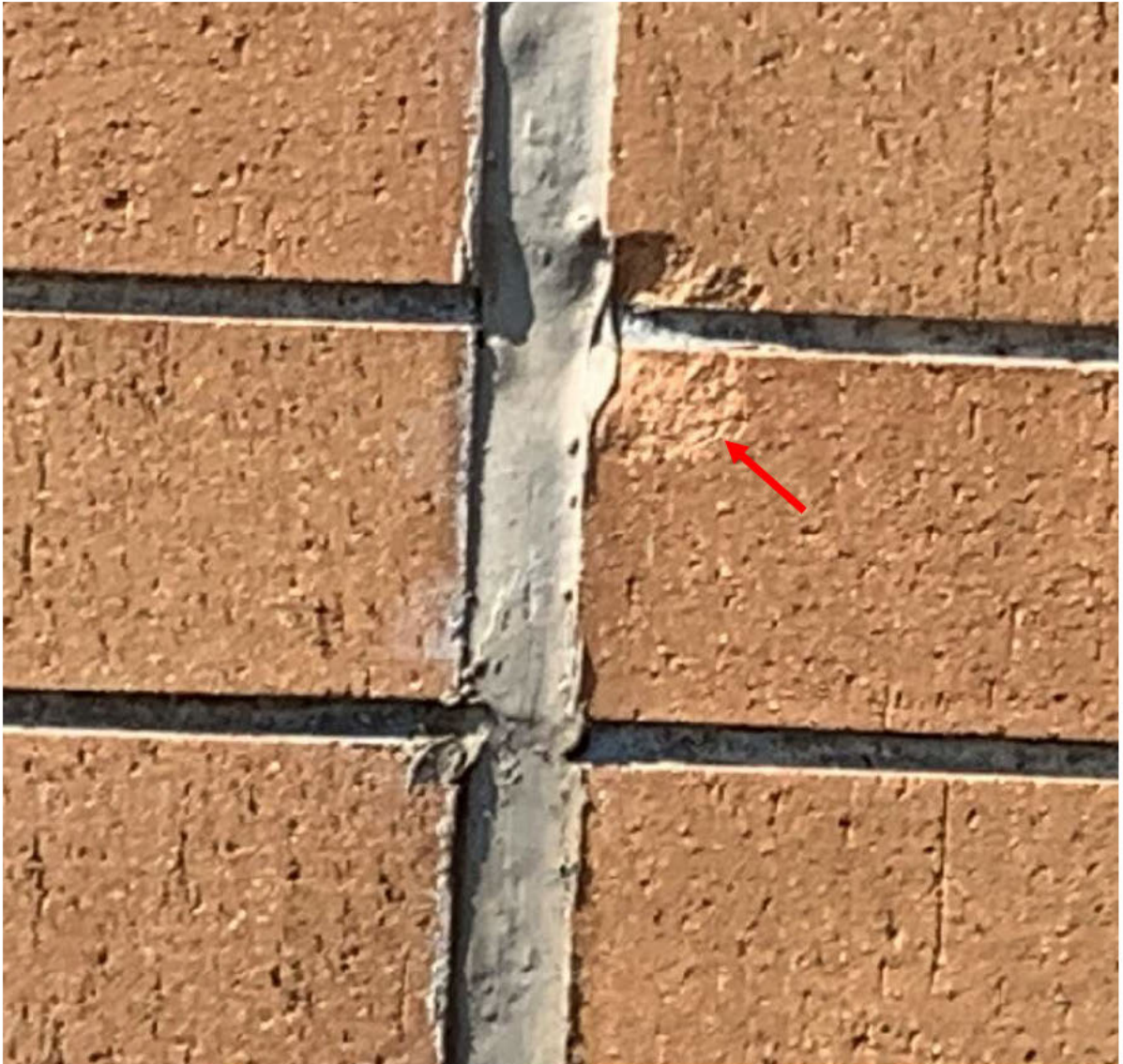
Figure 5: Spalling of brick masonry noted at Panel 205. Source: DeSimone.
