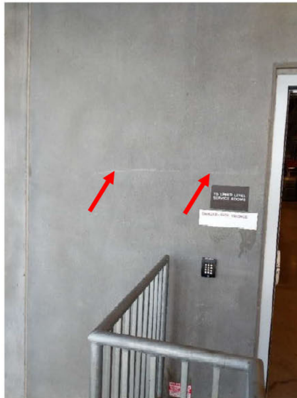
Figure 14: Repaired crack at exterior face of Panel 232. Source: DeSimone.
