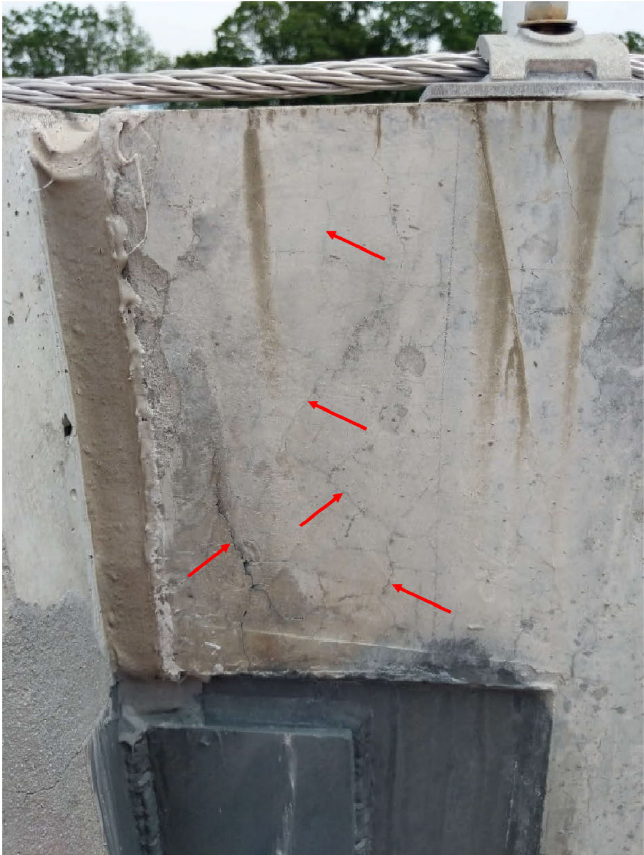
Figure 35: Spider cracks at interior of Panel WP-1328-RI. Source: DeSimone.
