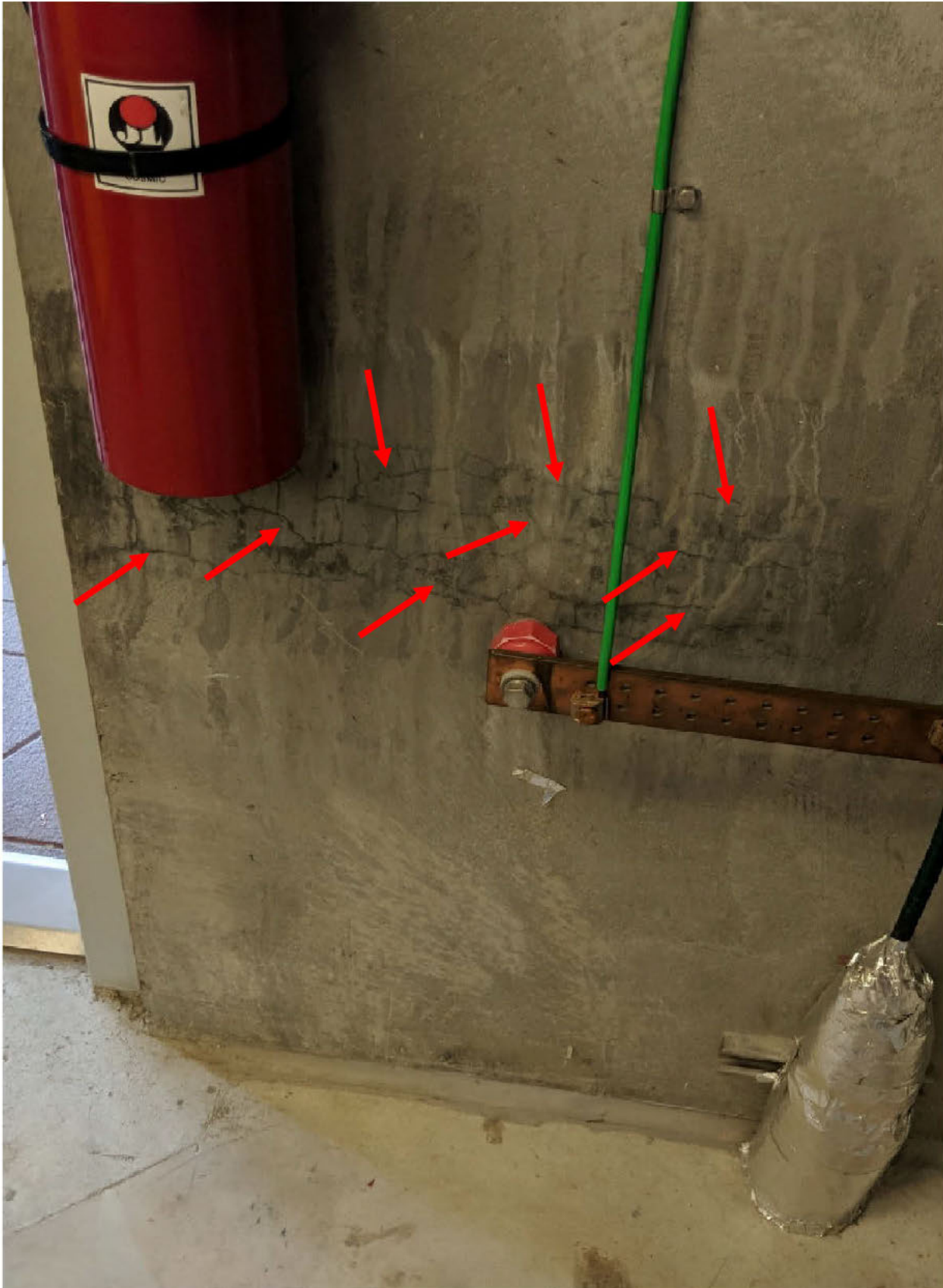
Figure 49: Spider cracks at interior face of Panel WP-1239. Source: DeSimone.
