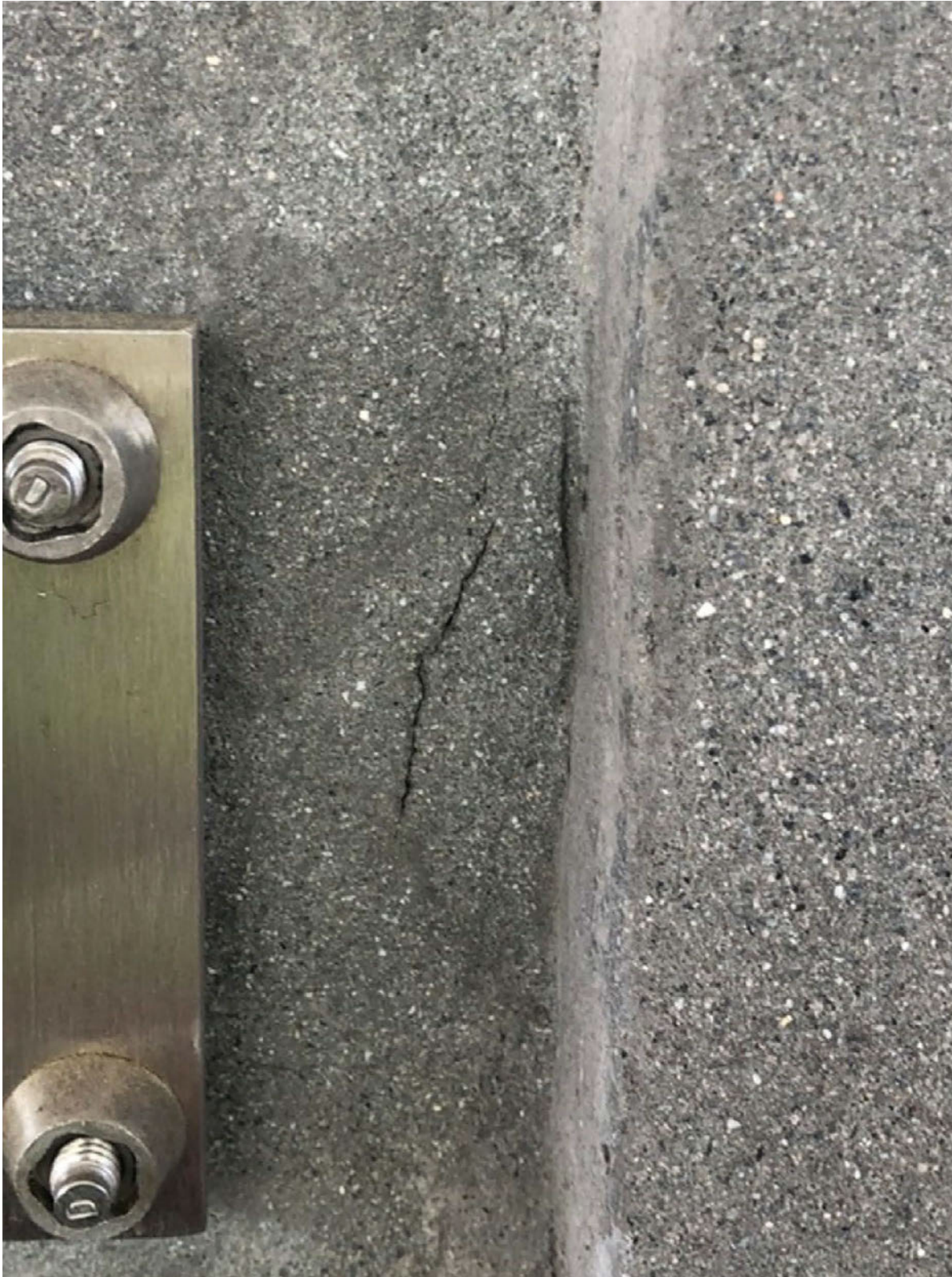
Figure 47: Crack at interior face of Panel WP-1233. Source: DeSimone.
