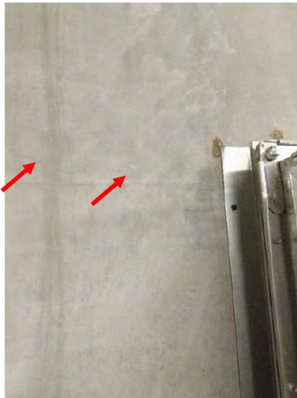
Figure 12: Crack at interior of Panel 219. Source: DeSimone
