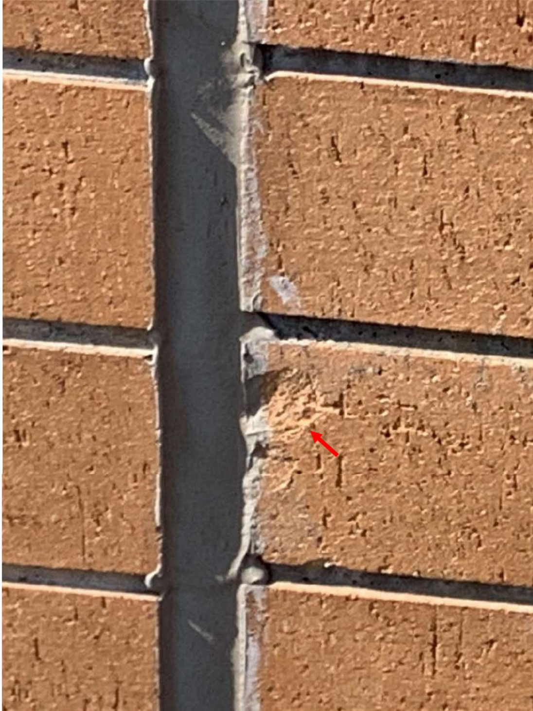
Figure 6: Spalling of brick masonry noted at Panel 219. Source: DeSimone.
