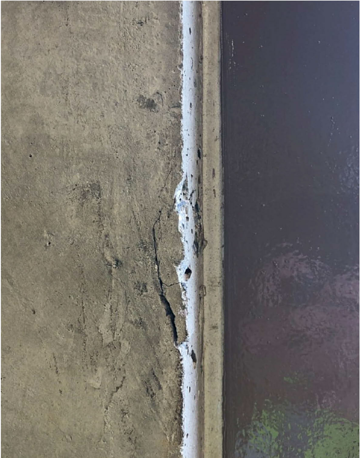
Figure 26: Chipped concrete at interior face of Panel 1420. Source: DeSimone.
