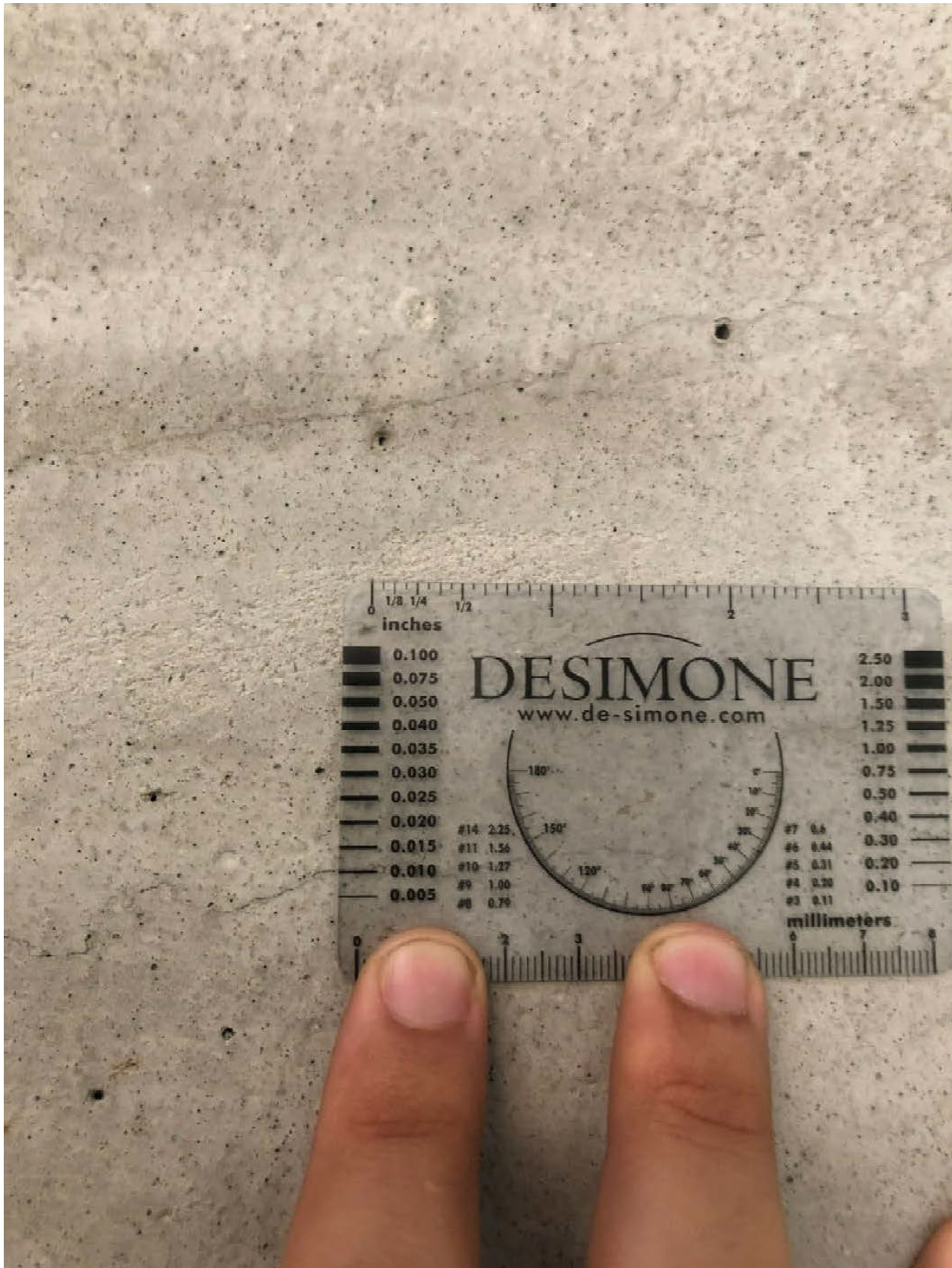
Figure 25: Crack at interior face of Panel 1421. Source: DeSimone.
