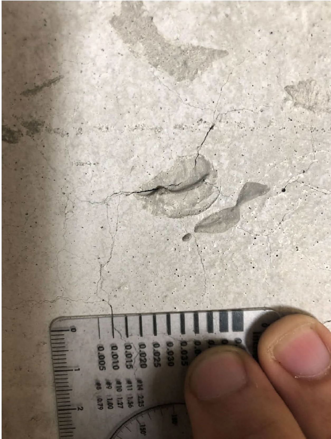
Figure 30: Crack at interior face of Panel 1904. Source: DeSimone.
