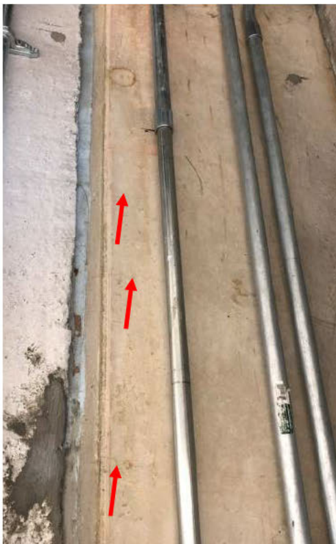
Figure 26: Interior face of Panel 1421 (Four cracks at this panel). Source: DeSimone.
