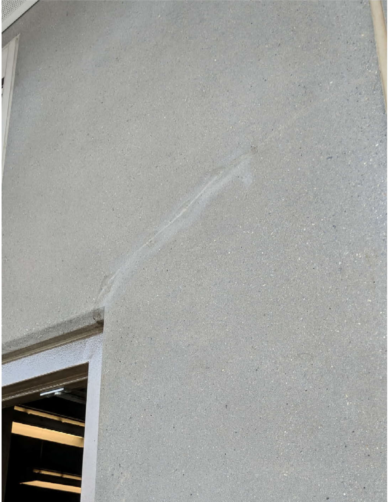
Figure 16: Repaired crack at exterior face of Panel 404. Source: DeSimone.
