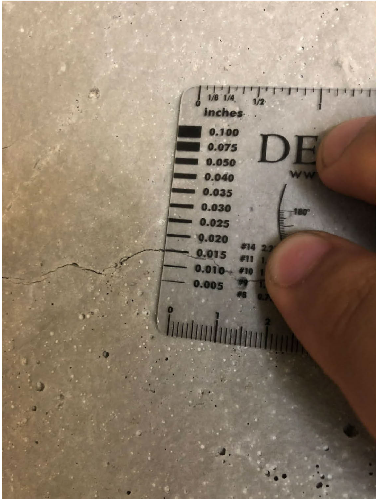
Figure 32: Crack at Interior face of Panel 1904. Source: DeSimone.
