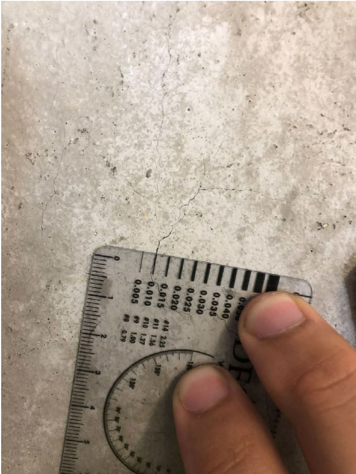
Figure 34: Crack at interior face of Panel 1904. Source: DeSimone.
