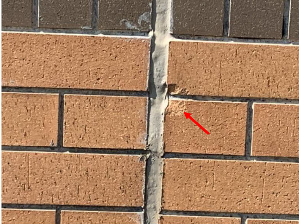
Figure 9: Spalling of brick masonry noted at Panel 205. Source: DeSimone.
