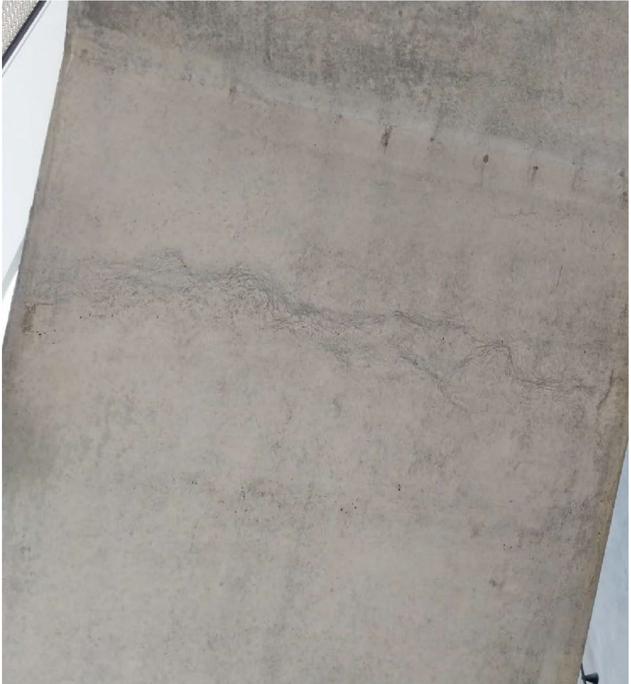
Figure 18: Crack at underside of Panel ST-4. Source: DeSimone.
