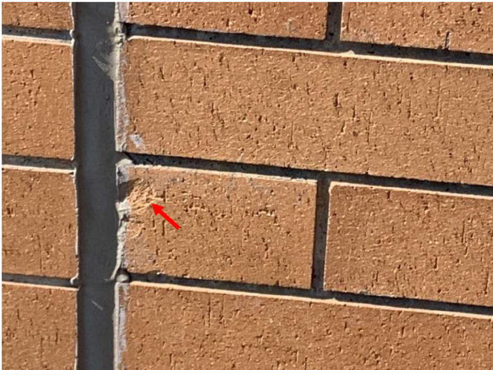
Figure 10: Spalling of brick masonry noted at Panel 219. Source: DeSimone.
