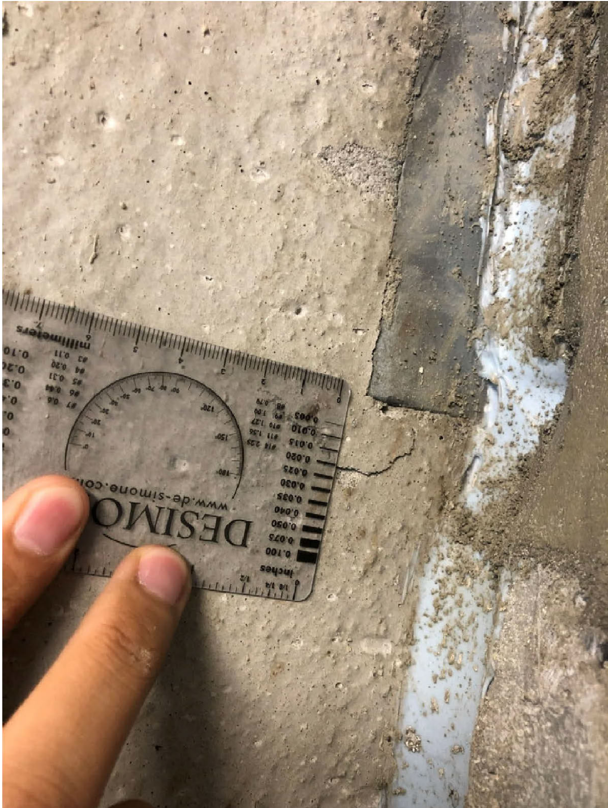
Figure 20: Crack at Interior face of Panel 1404. Source: DeSimone.
