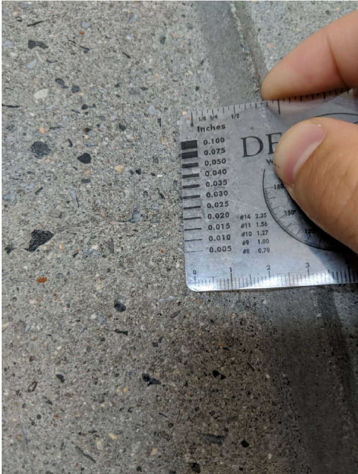
Figure 17: Crack at exterior face of Panel 107. Source: DeSimone.
