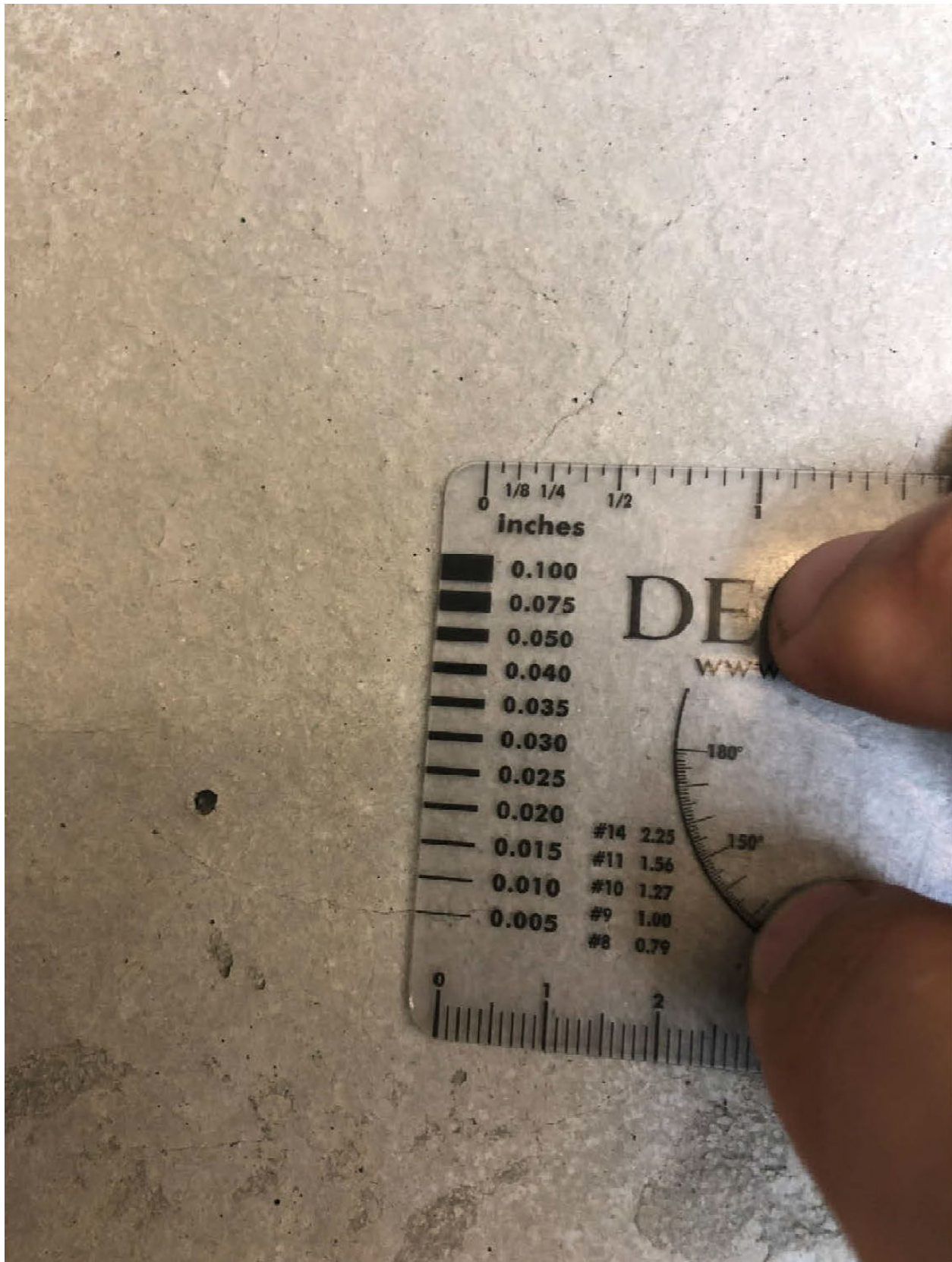
Figure 29: Crack at interior face of Panel 1904. Source: DeSimone.
