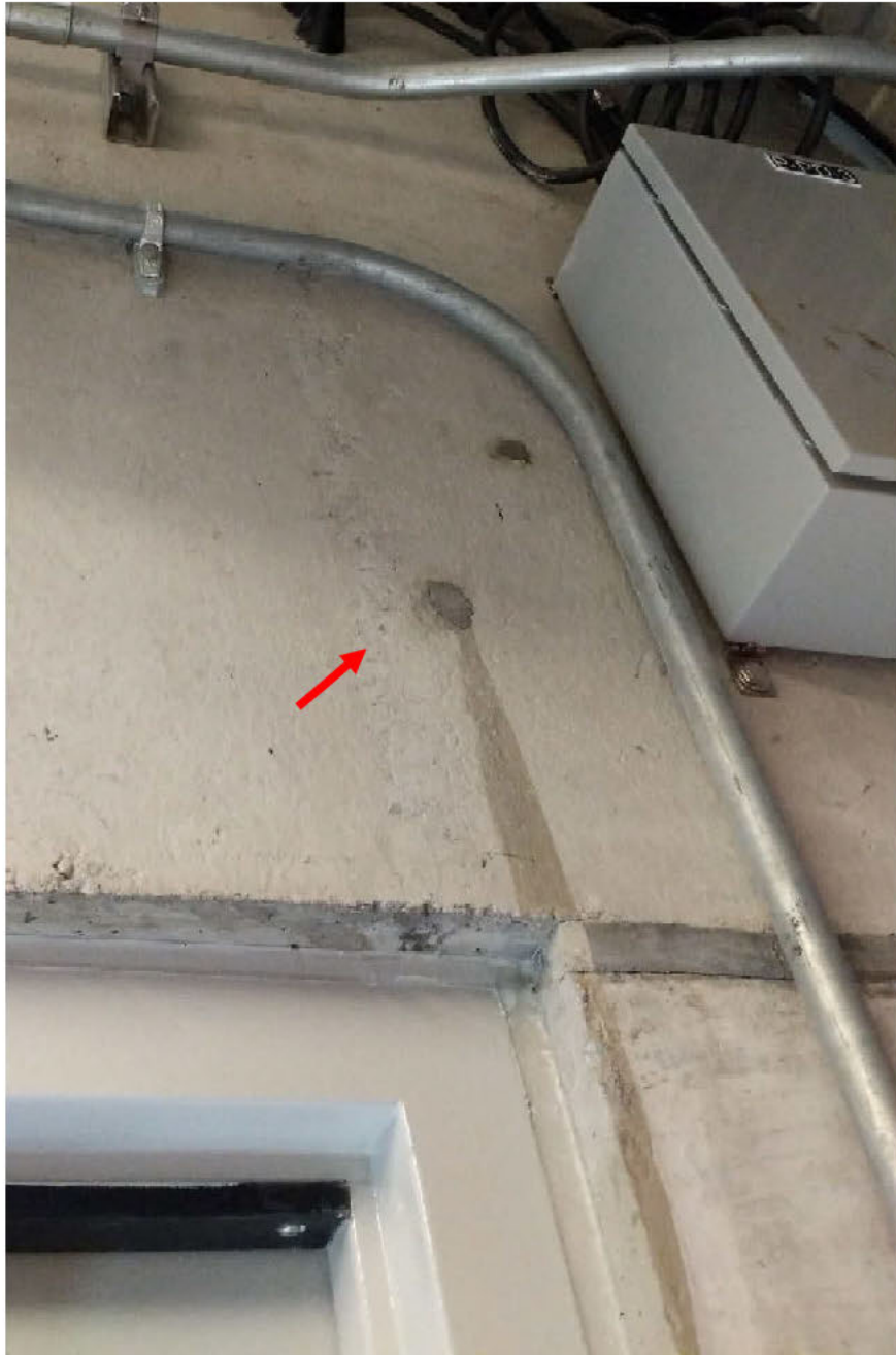
Figure 2: Efflorescence observed at Panel 100. Source: DeSimone.
