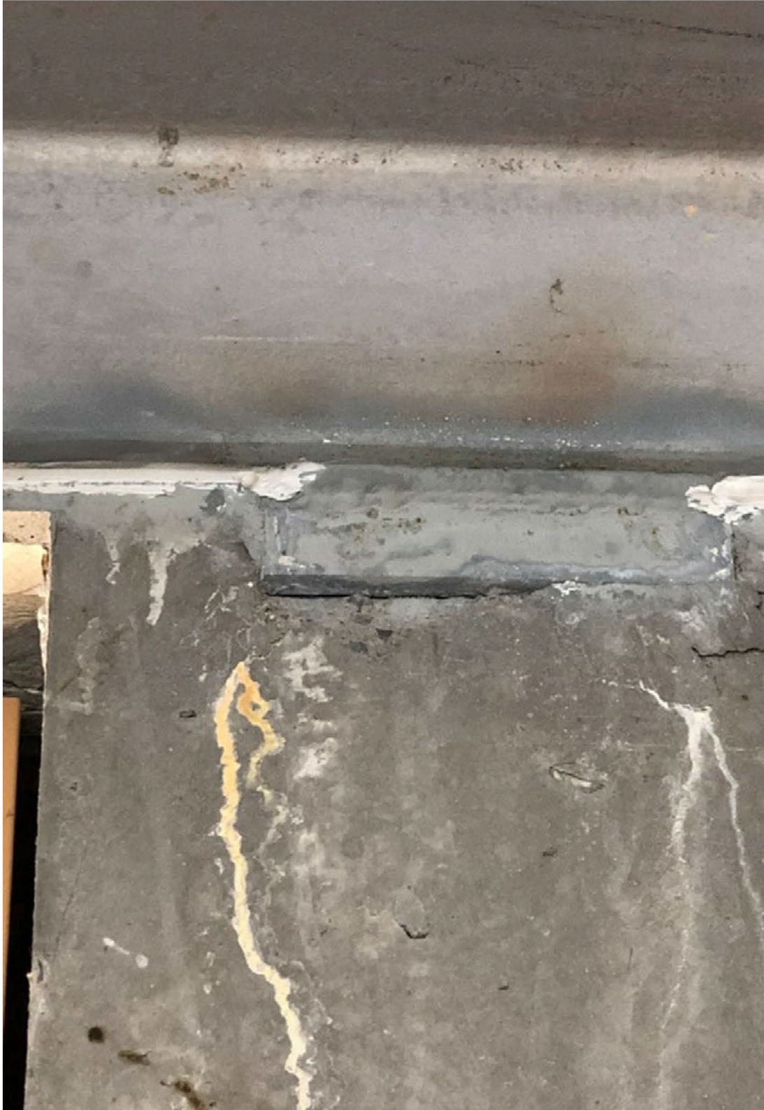
Figure 27: Chipped concrete at interior face of Panel 1901. Source: DeSimone.
