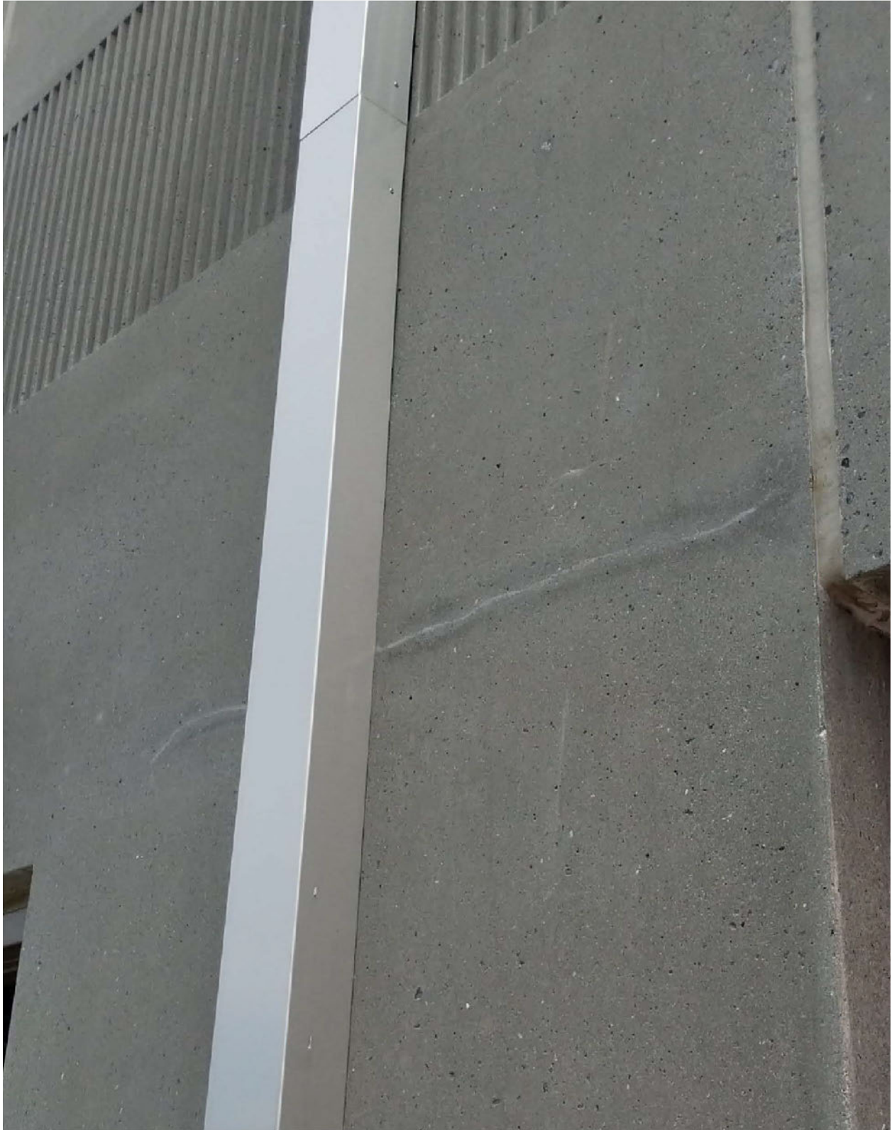
Figure 39: Previously repaired crack at exterior face of Panel WP-1313. Source: DeSimone.
