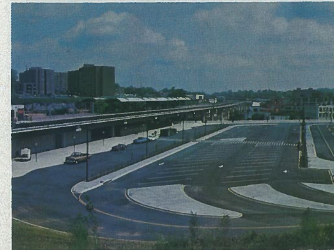
Rhode Island Avenue Station is the only station in Phase I that is aerial. The other four operating stations are subway.
