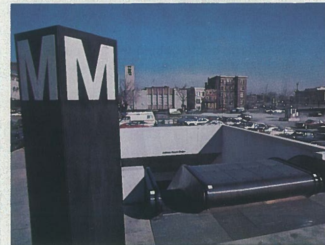
Stations are classified as either subway, surface or aerial. There are no surface stations in Phase I.
