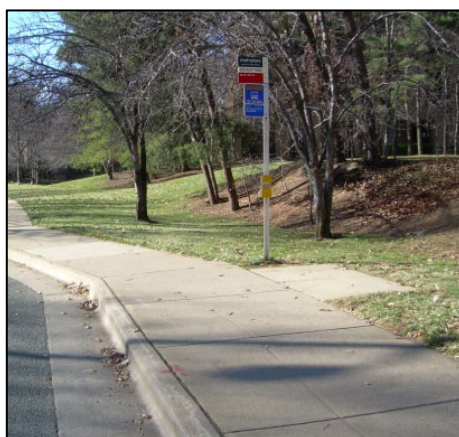
Landing pad on the backside of the sidewalk.
