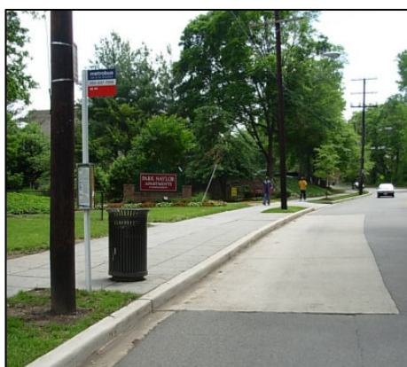
Expanded landing pad.
