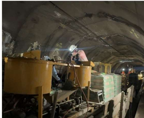
Water Leak Mitigation on Red Line
