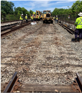
Track Repair at Takoma (Mud Spot Remediation)
