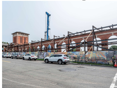
Historical Façade/Tower Bracing & Monitoring
