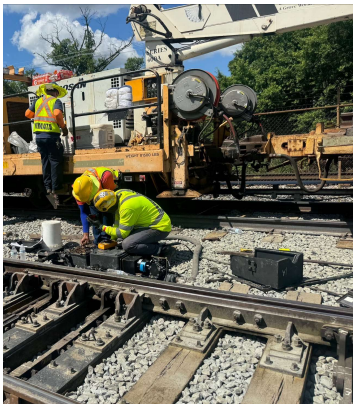
Switch Machine Replacement at Takoma
