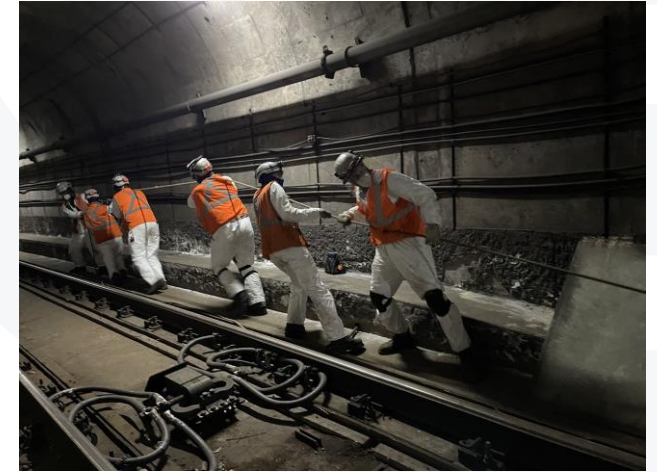
Cable Pulling at Rosslyn
