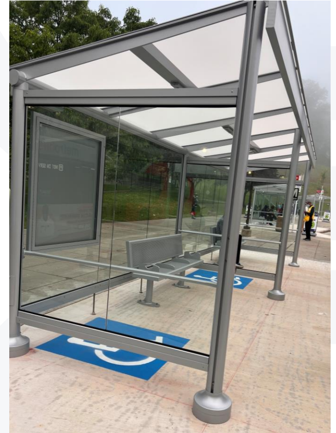
Fort Totten Station Bus Shelter
