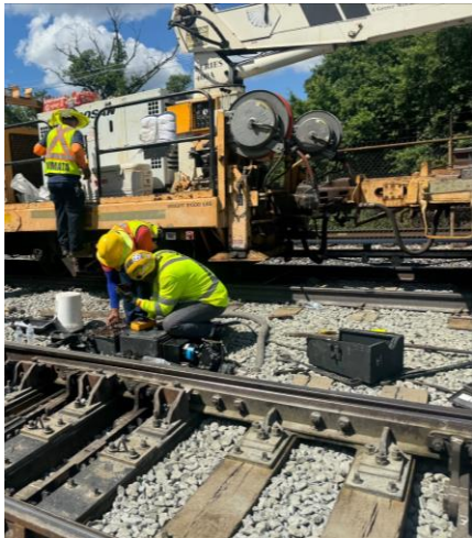
Switch Machine Replacement at Takoma
