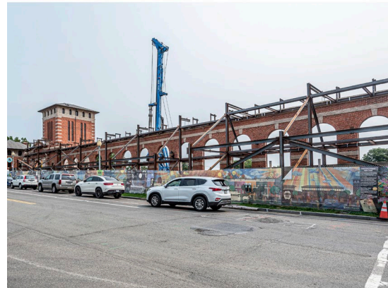
Historical Façade/Tower Bracing & Monitoring
