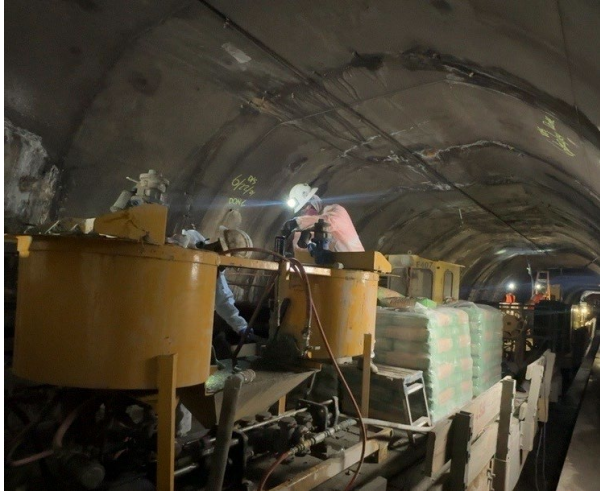
Water Leak Mitigation on Red Line
