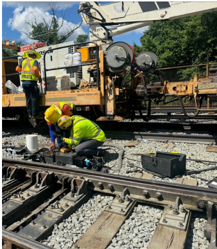
Switch Machine Replacement at Takoma
