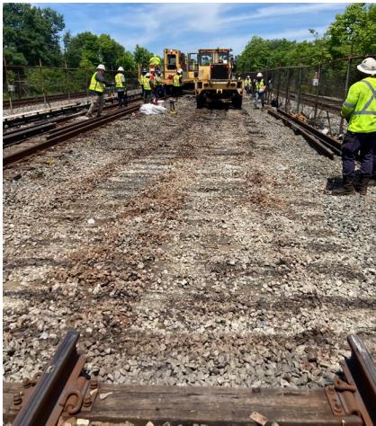
Track Repair at Takoma (Mud Spot Remediation)
