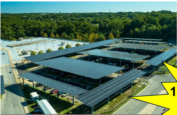
Southern Avenue Station
