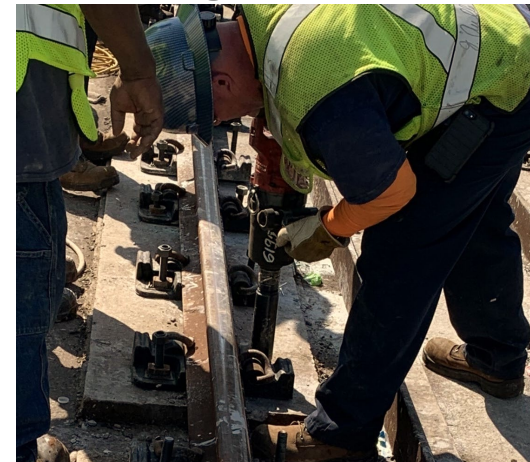
Installing Fasteners
