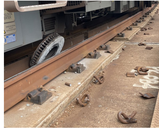
Installing Fasteners
