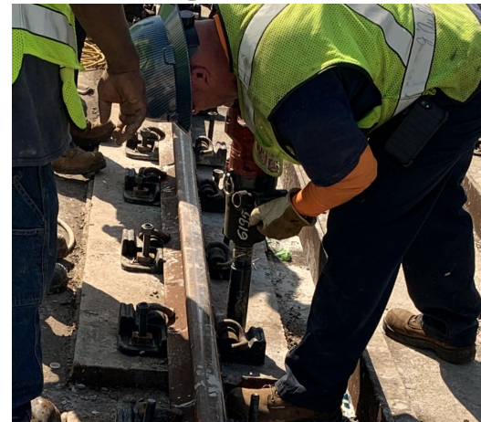
Installing Fasteners
