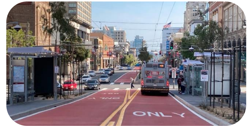
Center-running bus lanes: Van Ness St, San Francisco
