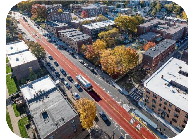
Center-running bus lanes, Columbus Ave, Boston
