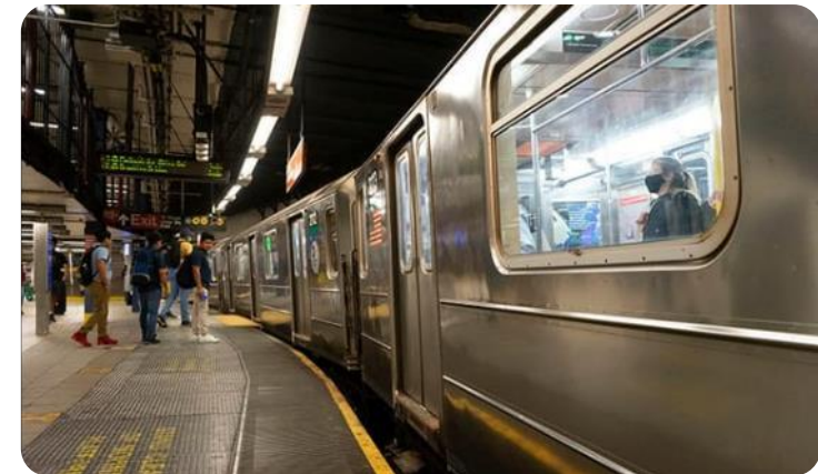
Train gaps at curved platform: 14 th Street-Union Square Station, New York
