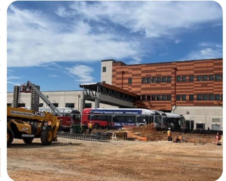
Bladensburg Bus Garage Construction
