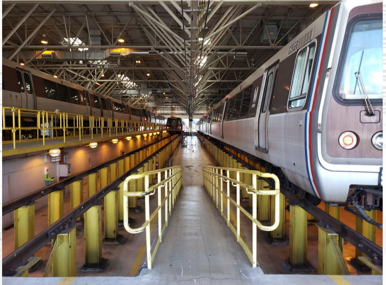
Shady Grove posted rail maintenance bay
