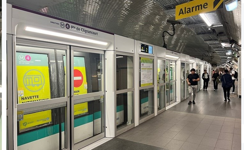
Paris Metro: Line 4 Platform Screen Door Testing
