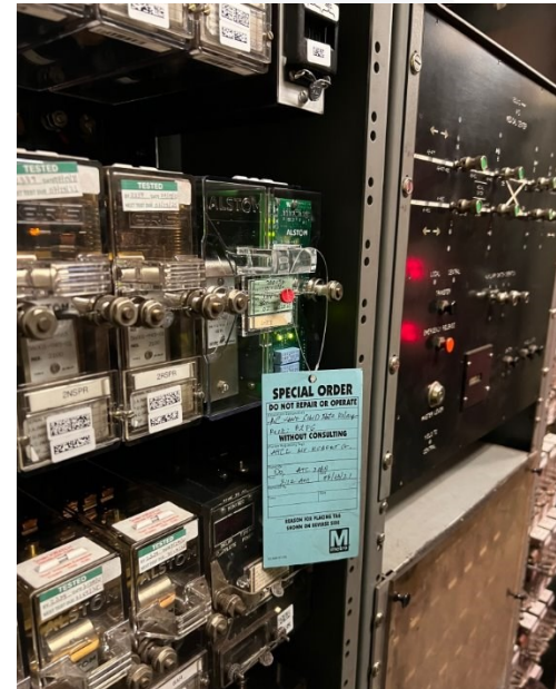
Vital Relays and Local Control Panel
