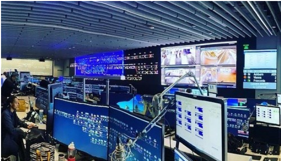
Metro Integrated Command & Communications Center (MICC)
