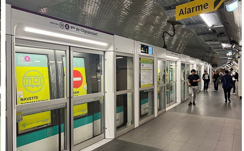
Paris Metro: Line 4 Platform Screen Door Testing
