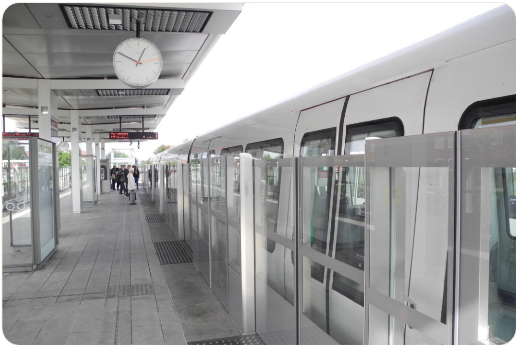
Kastrup Station, with platform screen doors – 2015
