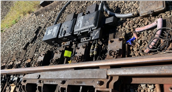
Signaling Switch Machine Replacement
