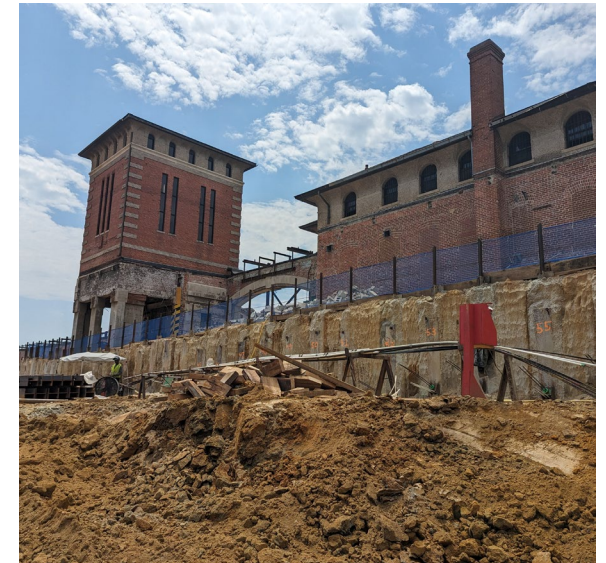
Two Bus Garage Groundbreakings
