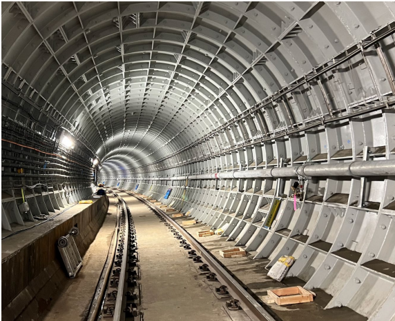
Yellow Line Tunnel Rehabilitation
