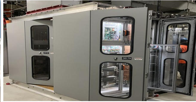
Traction Power Substation Replacement
