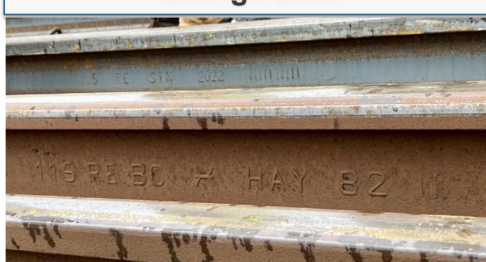
Rail Replacement – Orange Line
