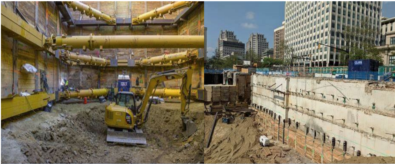
Ongoing Purple Line Construction at Bethesda
