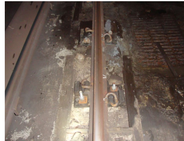
Deteriorated Grout Pad
