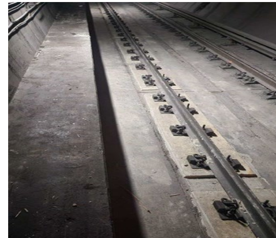
Restored Grout Pad
