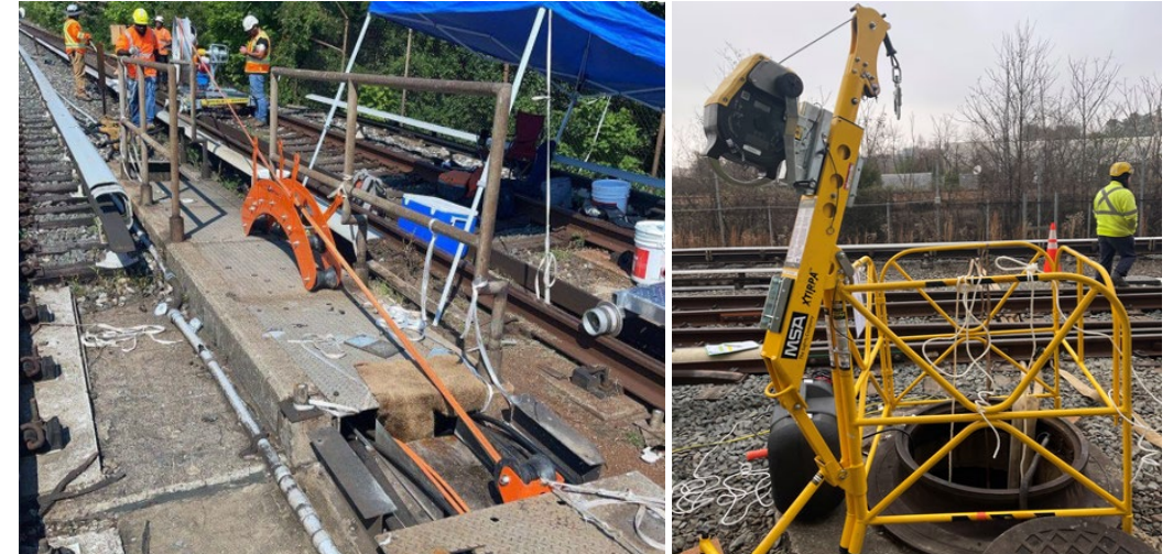
Fiber Installation Between Tracks and In Manholes
