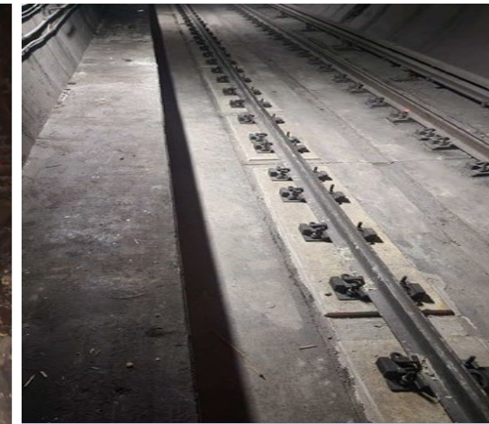
Restored Grout Pad
