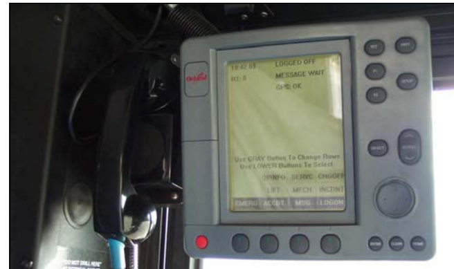
Automatic Vehicle Location/Bus Radio System Installation
