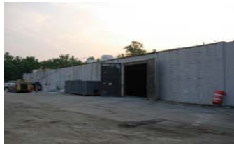
Salt Storage Facility
