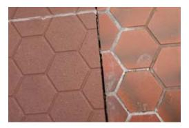
Testing has shown that the new precast concrete paver tiles are the most economical solution for Metrorail station floors and platforms. The tiles have proven to be more durable, which will result in lower maintenance costs. They are also not as slick when wet.
