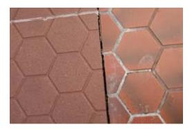
Testing has shown that the new precast concrete paver tiles are the safest and most economical solution for Metrorail station floors and platforms. The tiles have proven to be more durable, which will result in lower maintenance costs. They are also not as slick when wet.
