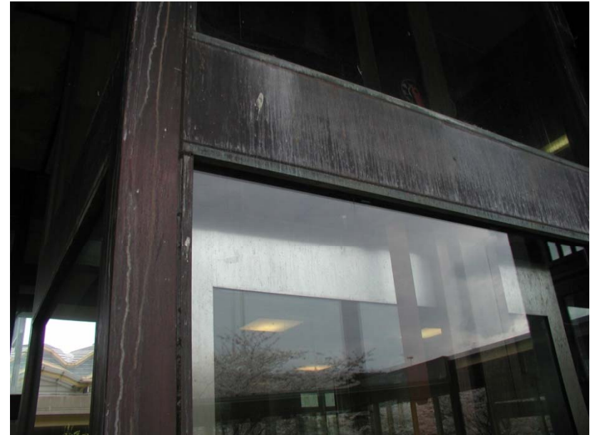
Rebronzing elevators, escalators, exterior pylons, and handrails
