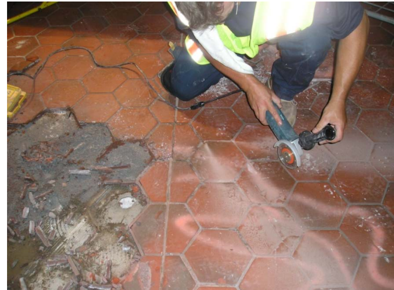
Replacing broken tiles
