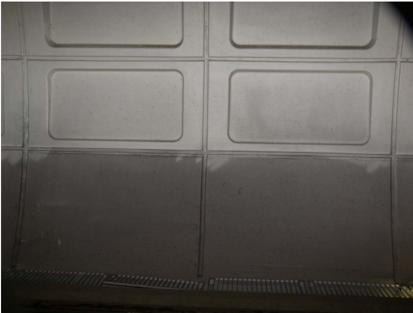
Cleaning station walls
