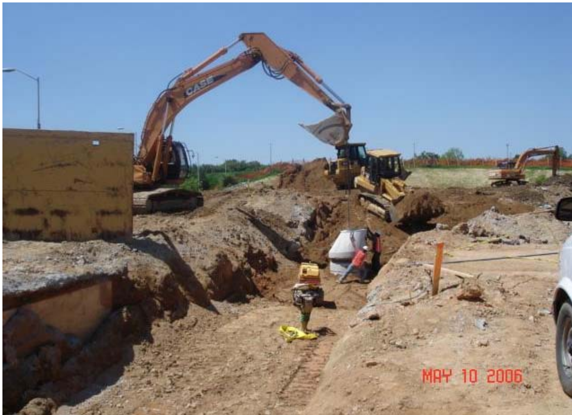
Placement of fill over the 78" storm water pipe.
