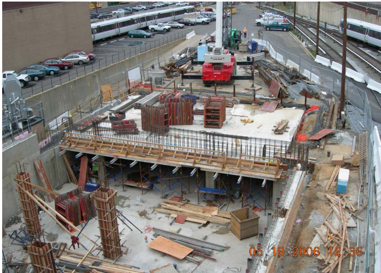
Construction of the new loading dock.
