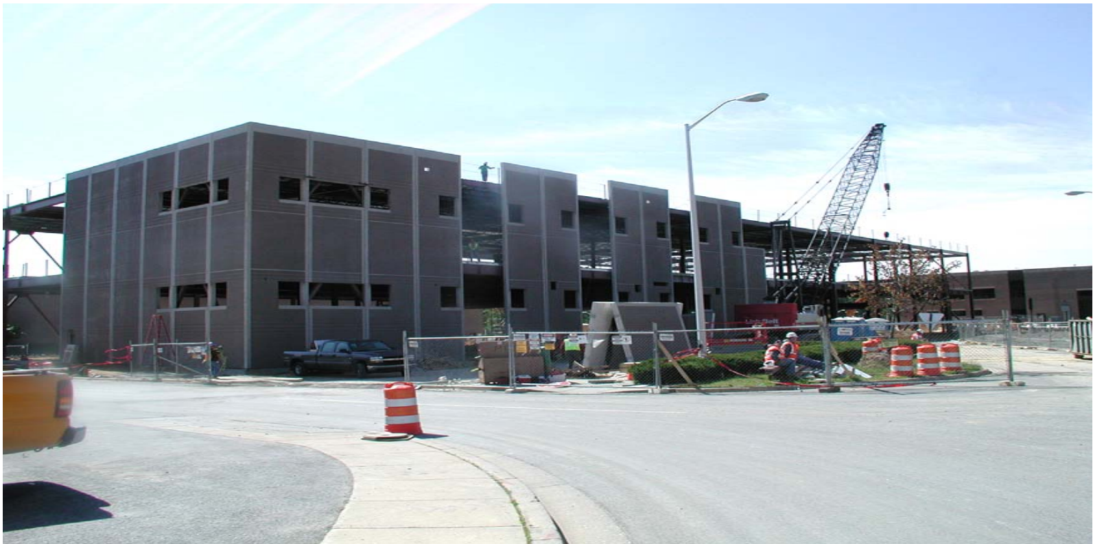
Pre-cast concrete installation for the annex.
