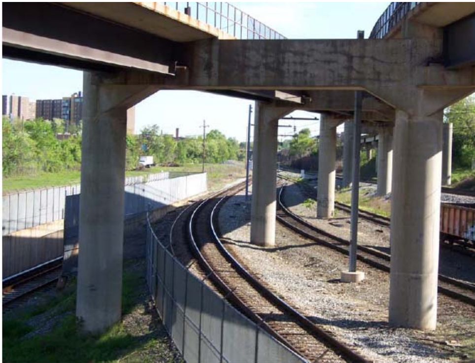
Rhode Island Avenue Aerial Structure – Pier Cap over CSX
