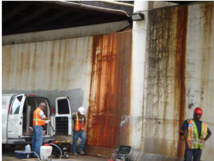
First Street Bridge South Abutment
