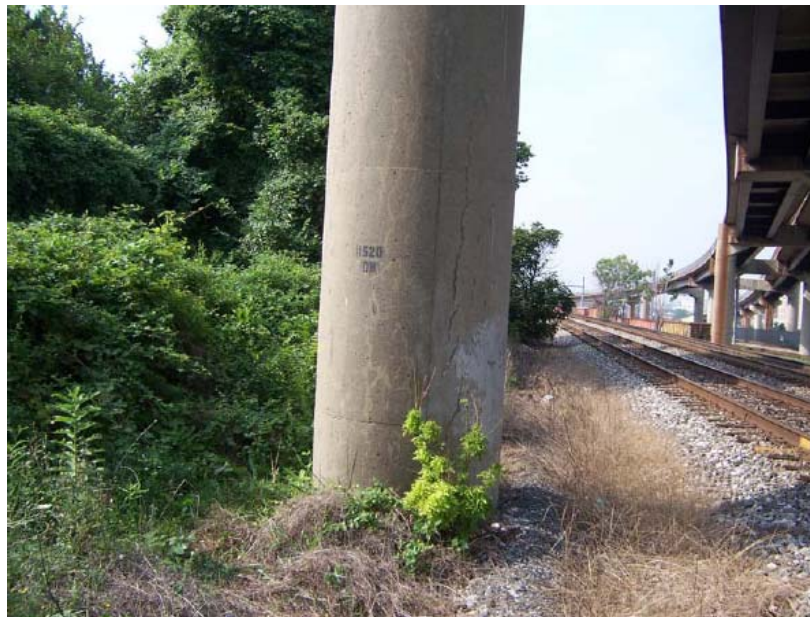
Rhode Island Avenue Aerial Structure
