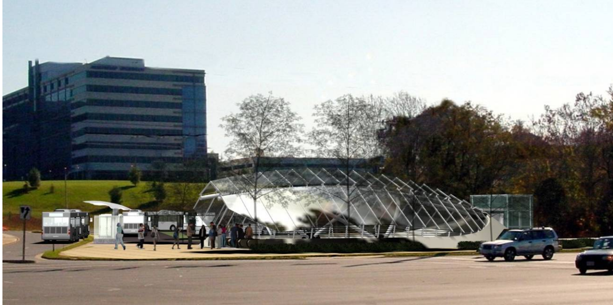
Figure 2. Tysons East Station Entrance is designed protect the patrons, the escalators and provide closure at the street level for security.
