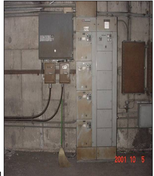
Motor Control Center prevents Damage to Motors due to Over/Under Voltage & Prevents Flooding/Poor Ventilation
