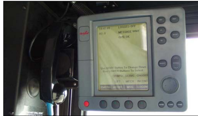
Automatic Vehicle Location/Bus Radio System Installation
